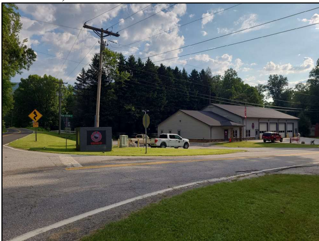
Figure 5: Manicured Lawn and Fire Department at West End of Project Area (Looking Northeast)
