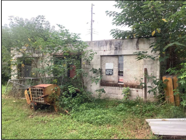
a. Oblique, Looking Southeast
