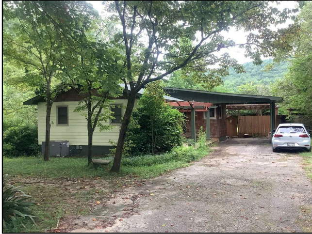
a. Oblique, Looking Southeast
