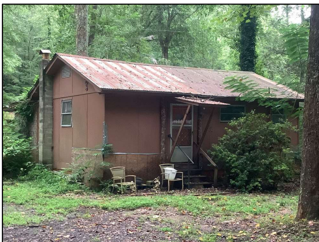
c. Oblique, Looking South
