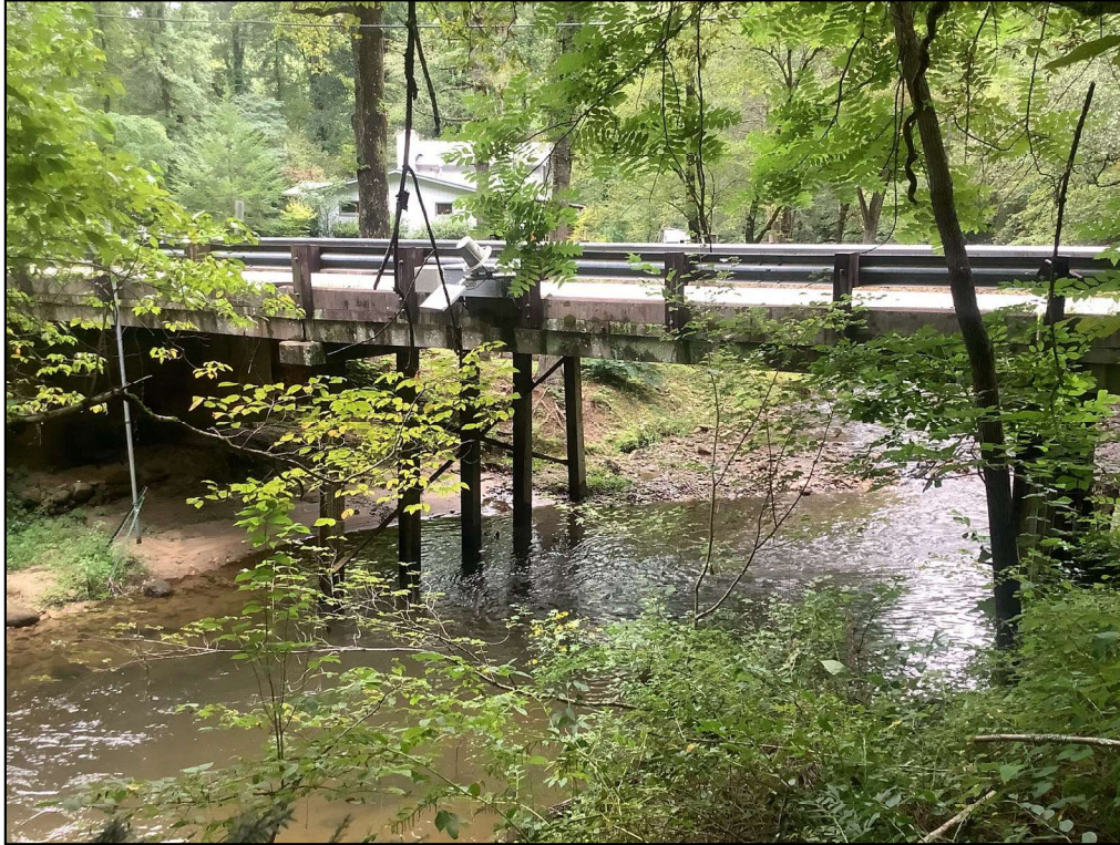
a. View of Bridge, Looking Northeast
