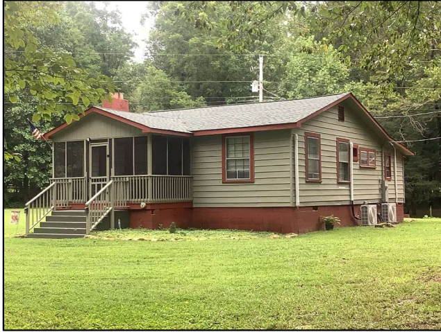
a. Oblique, Looking Northwest
