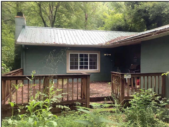
b. Entrance and Façade Detail, Looking Southeast
