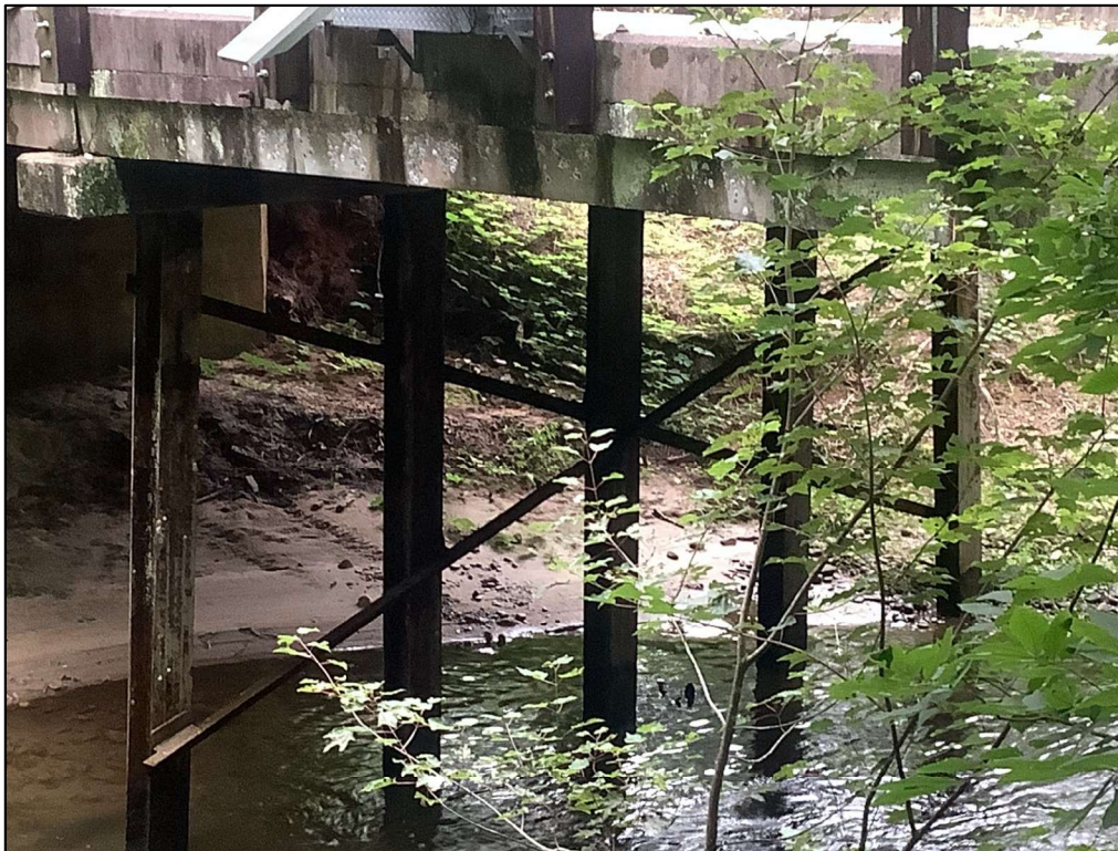
b. Bridge Structure, Looking Northeast
