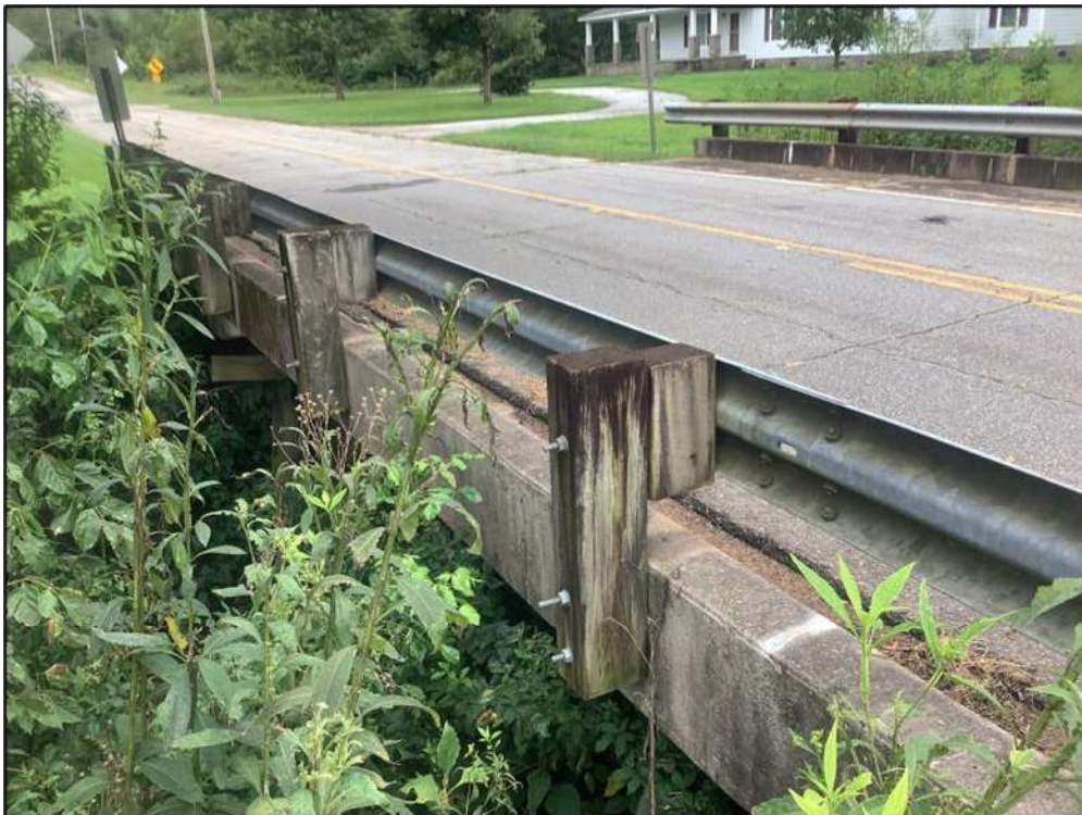
b. Southern Overflow Bridge (Built 1969), Looking Southwest
