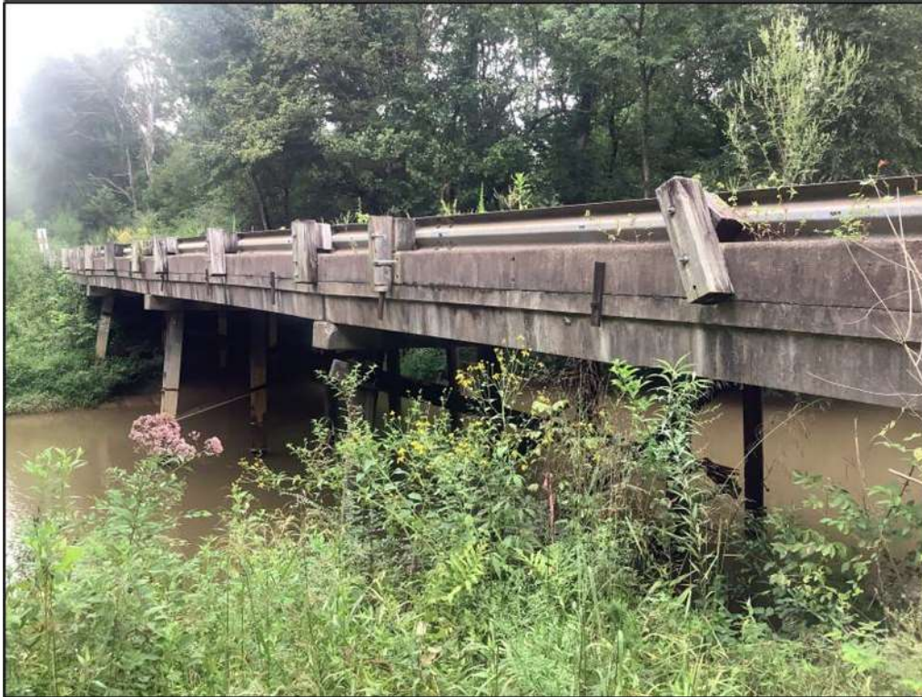
a. Bridge Structure, Looking Northeast
