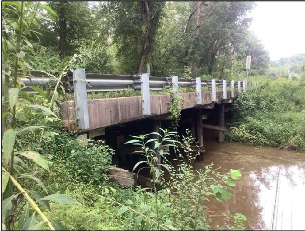
a. Northern Overflow Bridge (Built 1957), Looking Southeast
