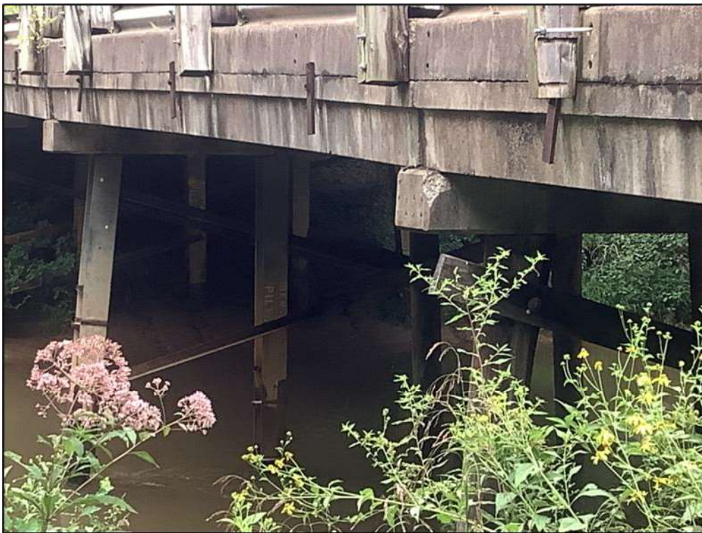
b. Bridge Structure Detail, Looking Northeast
