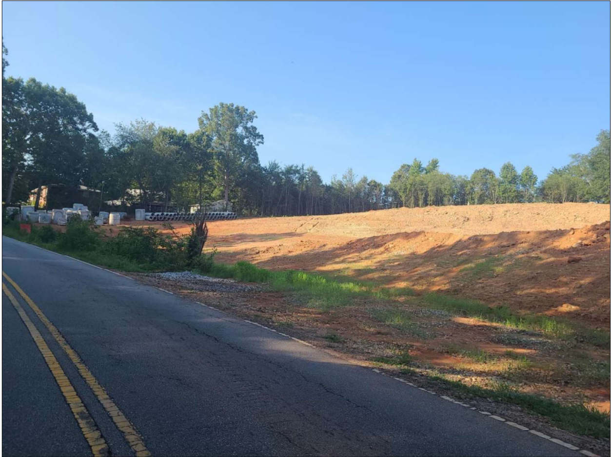
Figure 4. New Construction on West Side of Crestwood Drive, Looking South
