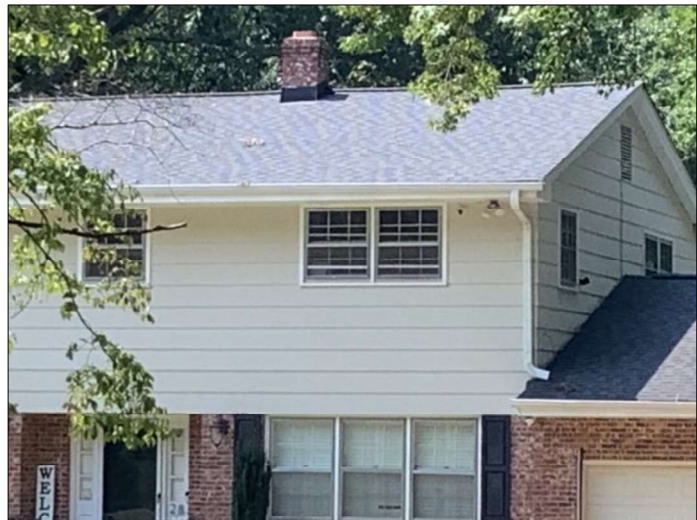
c. Façade Detail, Looking Southwest
