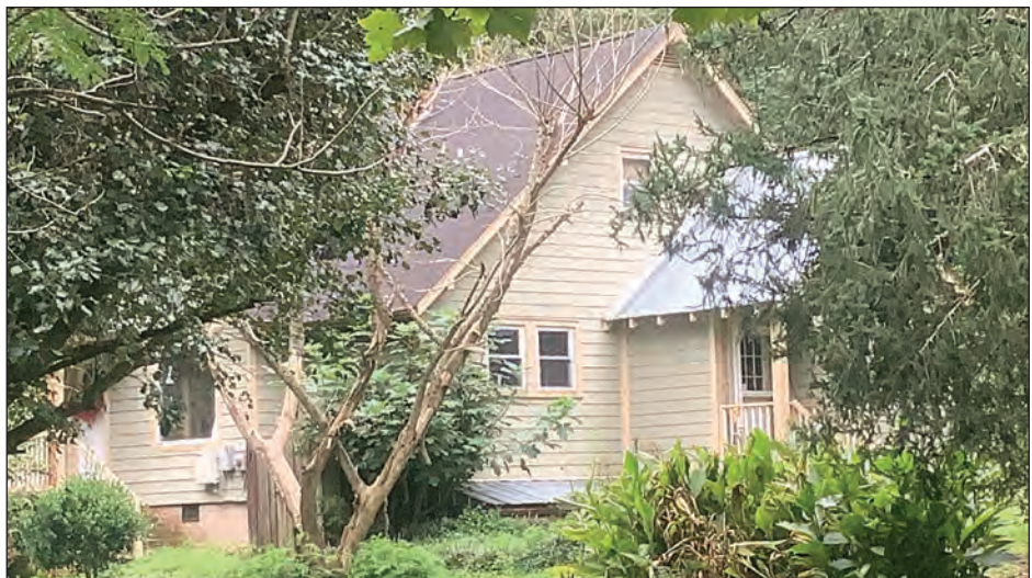
C. Oblique, Looking Northwest
