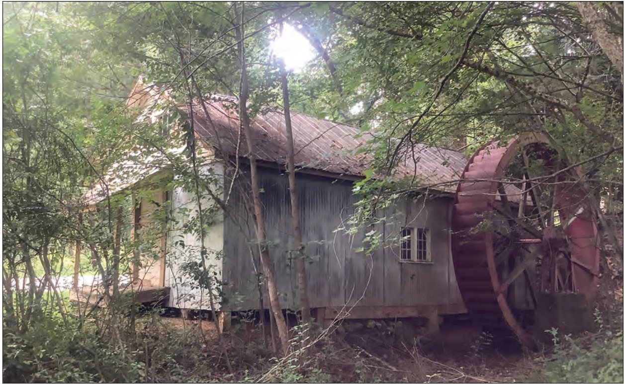
A. Oblique, Looking Northwest
