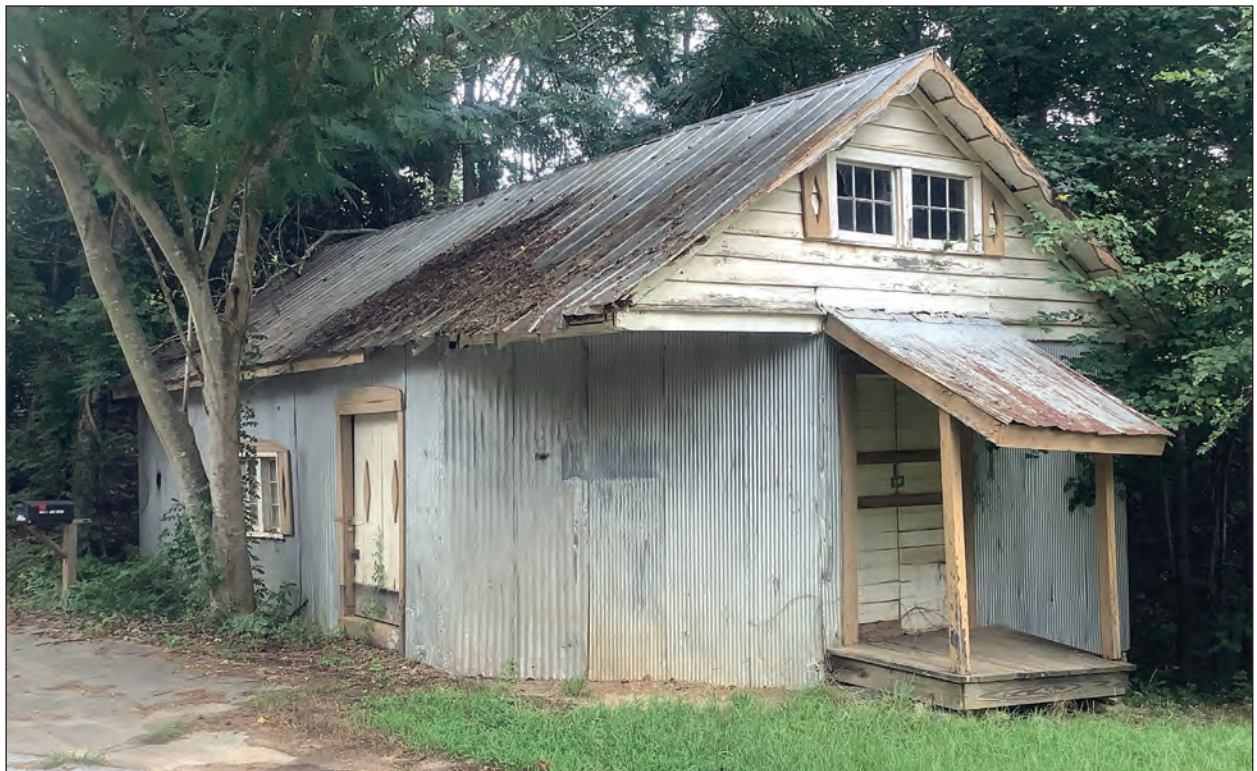
B. Façade, Looking North
