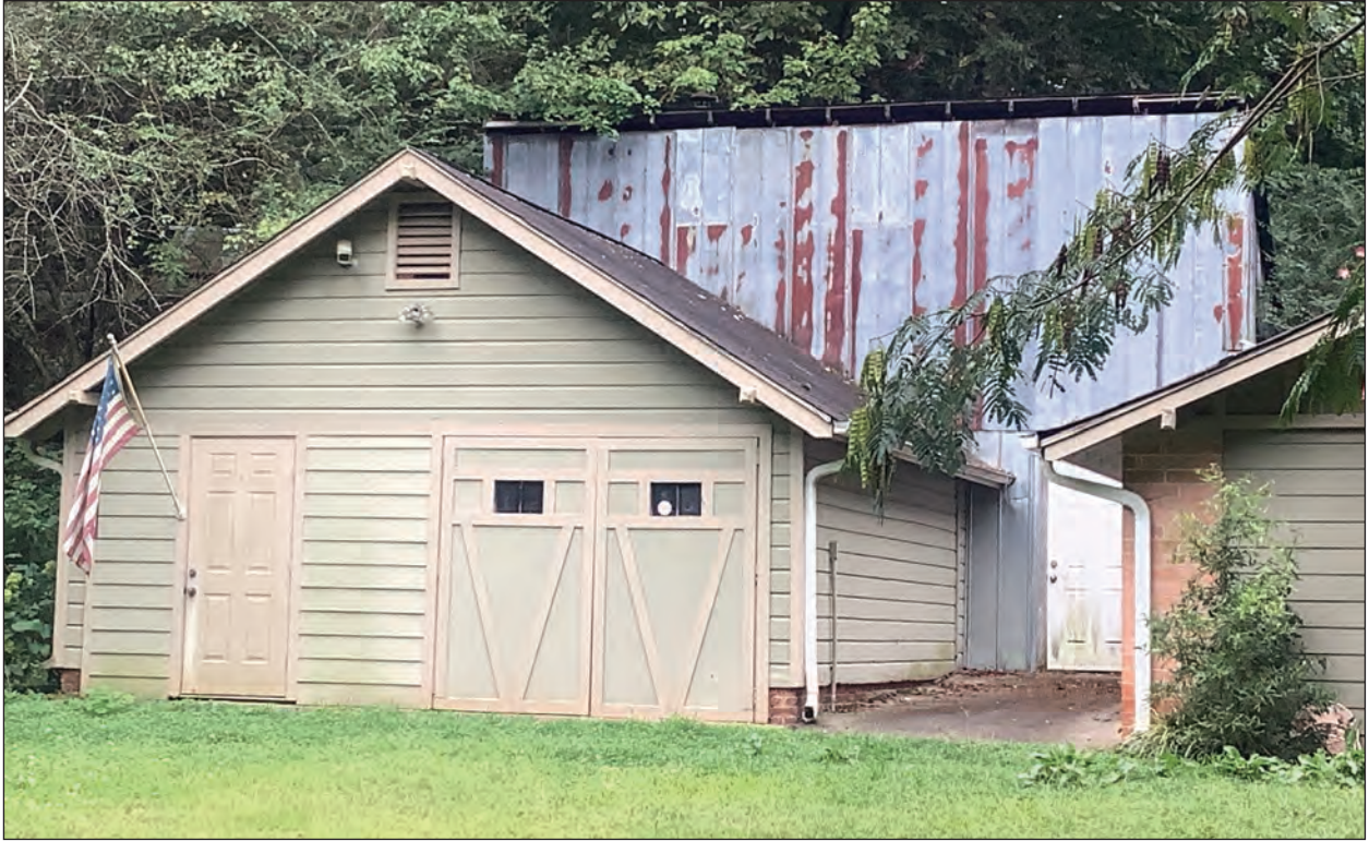
A. Oblique Showing Rear Addition, Looking Southwest
