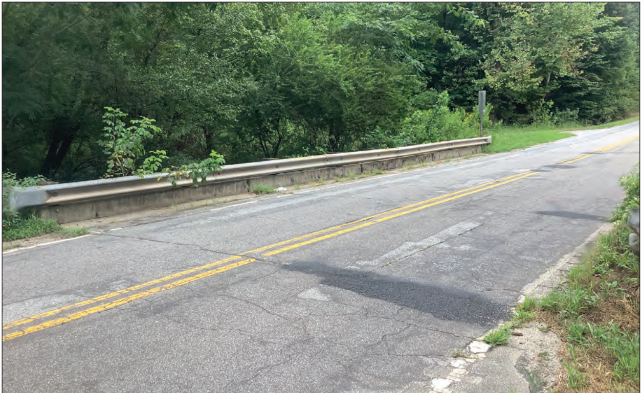
B. Bridge Surface, Looking Northeast
