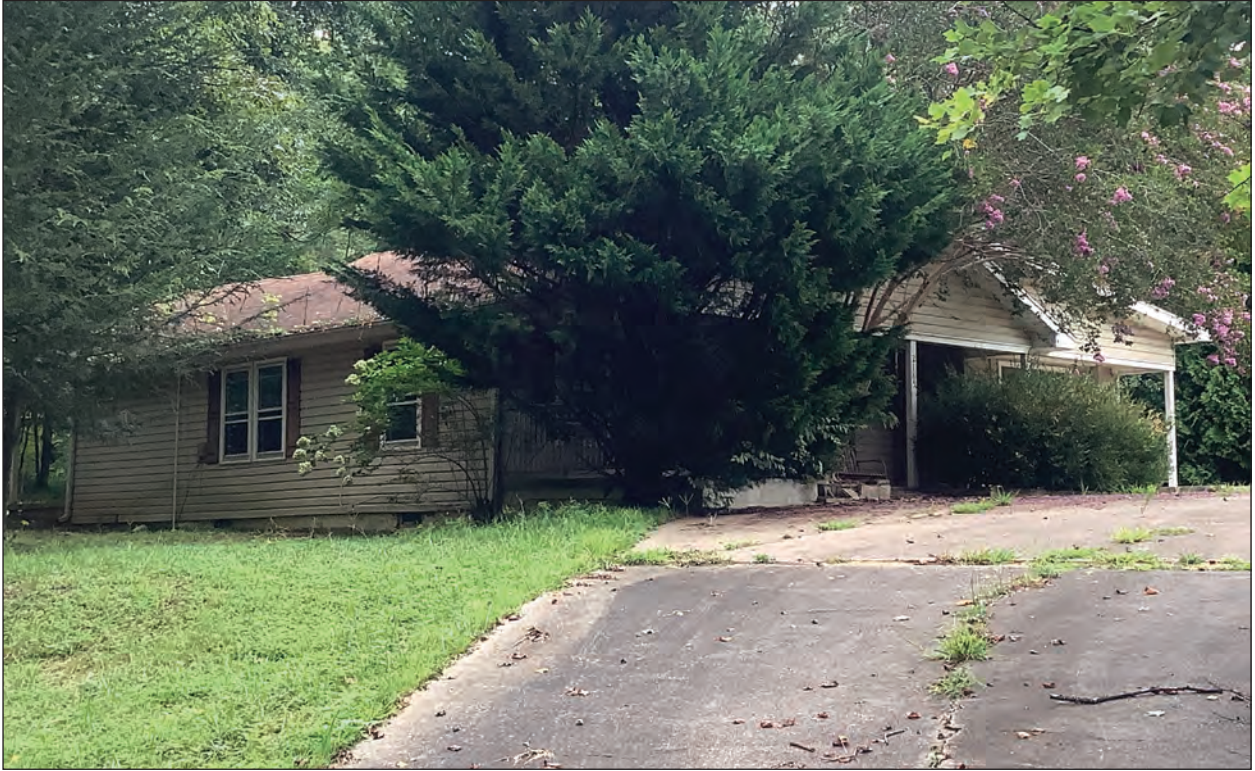
A. Oblique, Looking North
