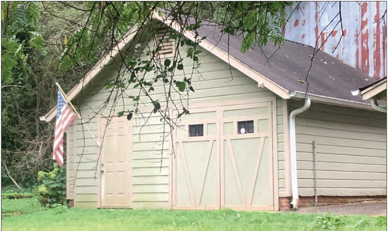
B. Oblique Detail, Looking Southwest
