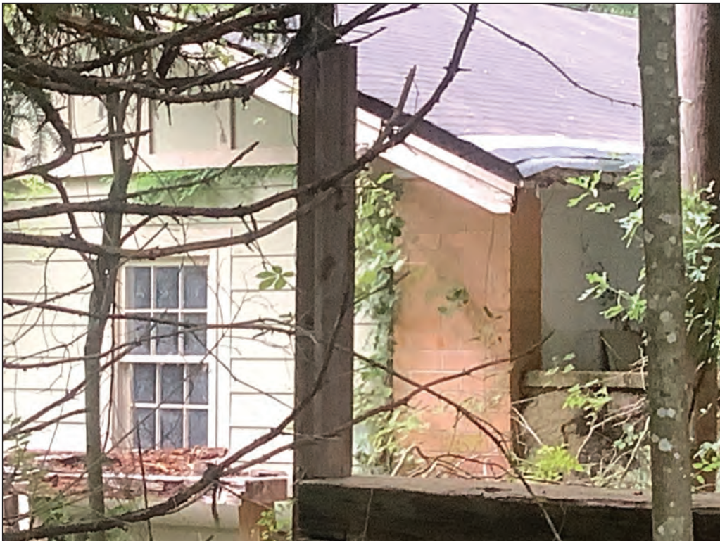
B. Oblique Detail, Looking Southwest
