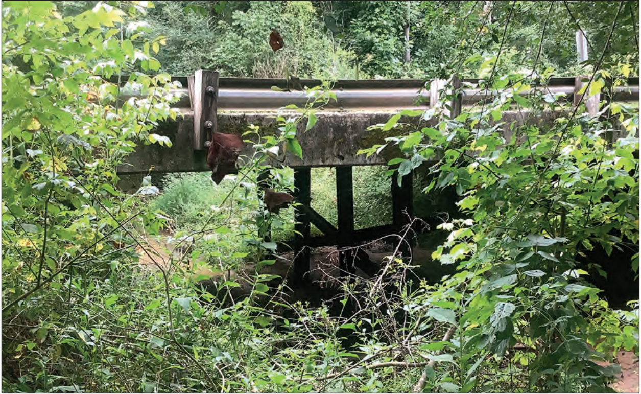
A. Bridge Structure, Looking Northeast
