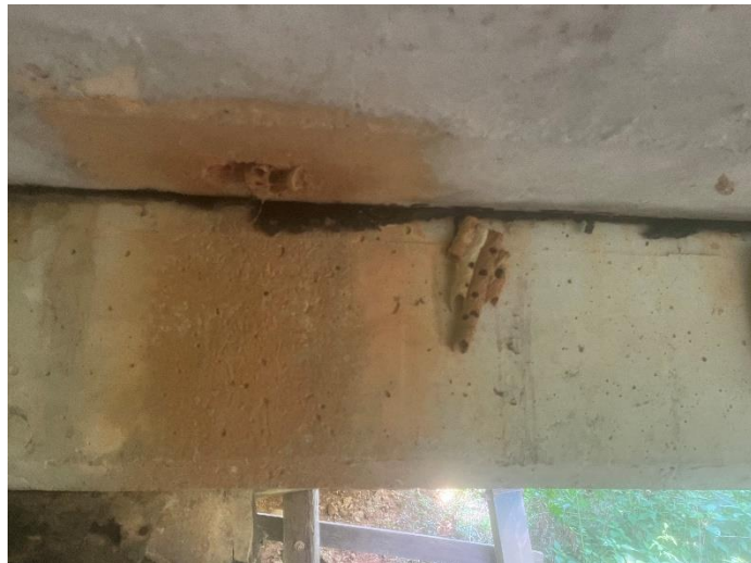
Photo 3: HA #2: Tar and Felt Vibration Dampener
