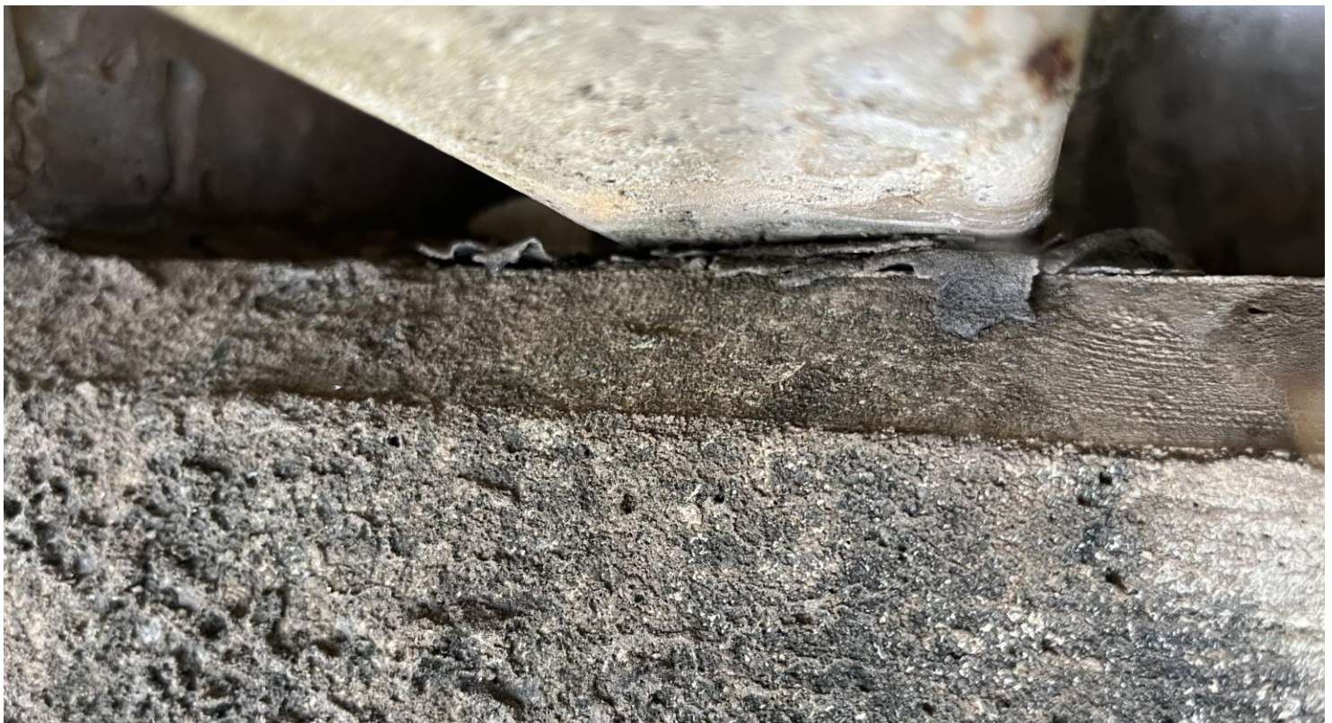
PHOTO # 4 View of HA #1 thin felt vibration dampener.
