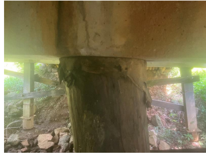
Photo 2: HA #1: Felt Vibration Dampener
