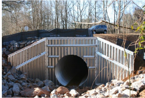
Use Pipe Wingwall
