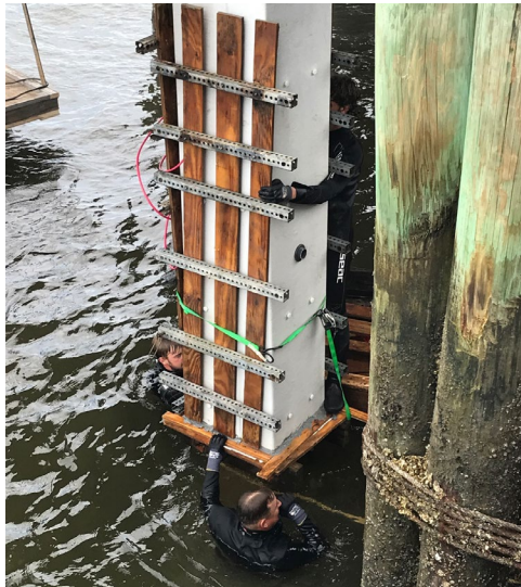
Pile Jackets on Ft Sumter Dock Rehabilitation installed by Cape Romain
