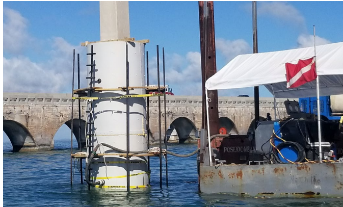
Pile Jackets in FL Keys designed by 3ePlus.
