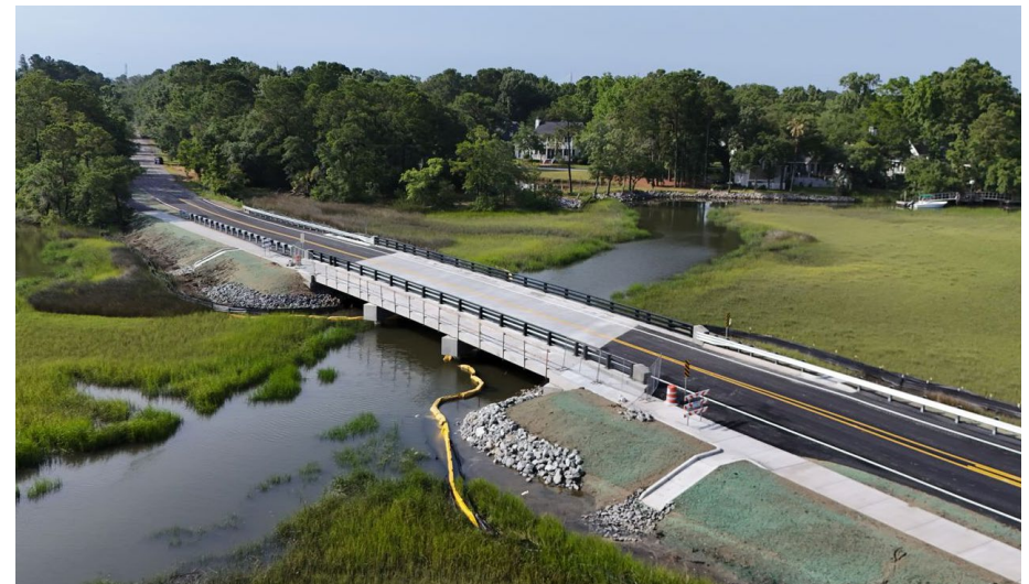
Beresford Creek Bridge, Charleston, SC First Bridge in SC with all GFRP Reinforcement
