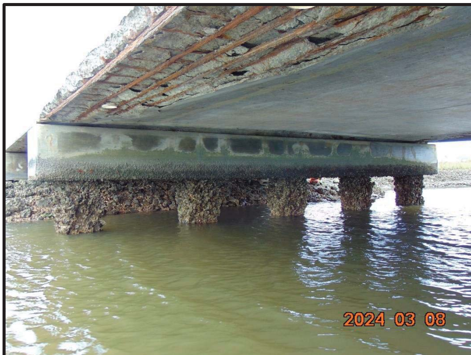
Photo 16: Bent 3 (Looking Upstream)
