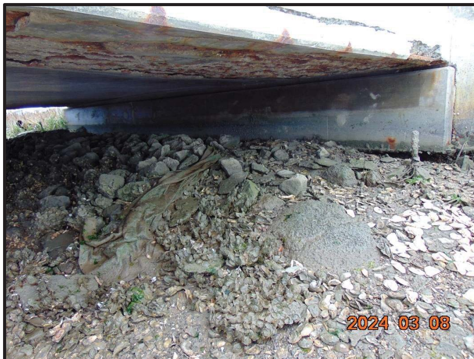
Photo 14: Bent 1 (Looking Upstream), Abutment 1
