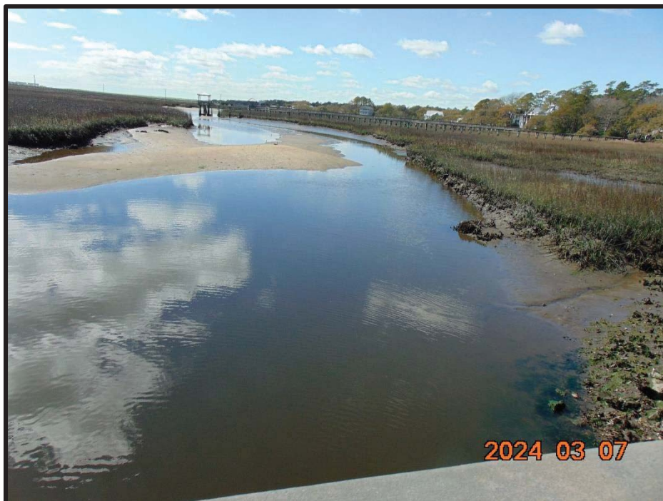
Photo 12: View From Bridge Deck (Looking Downstream)
