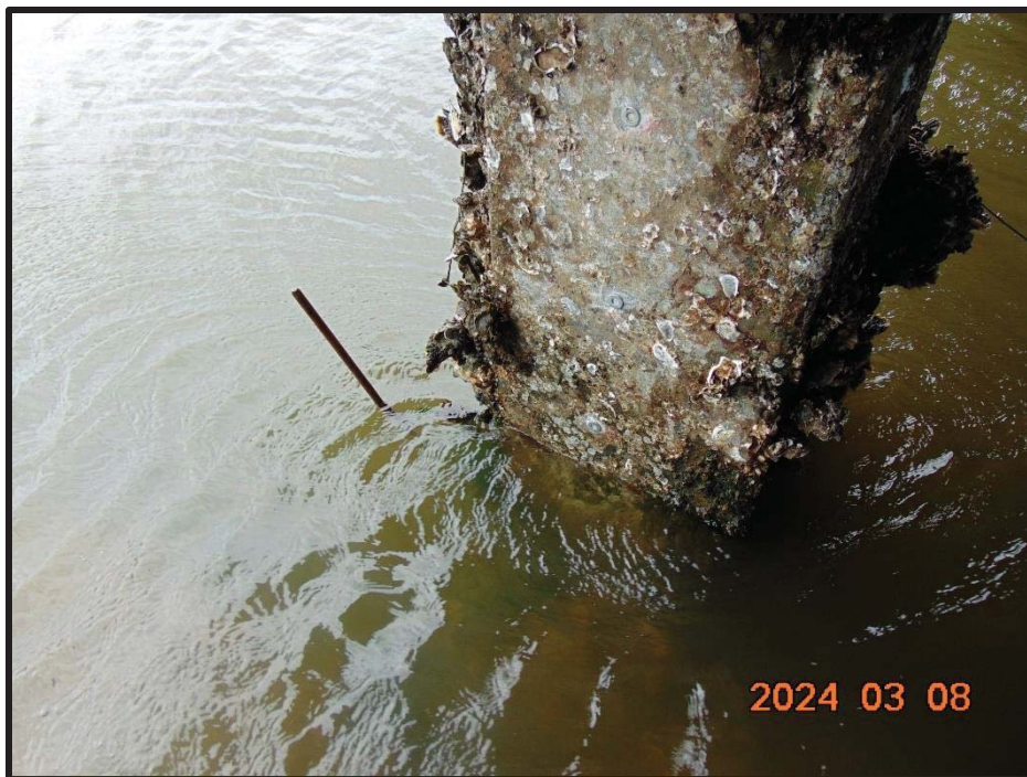
Photo 18: Substructure Bent Features Testing Probe
