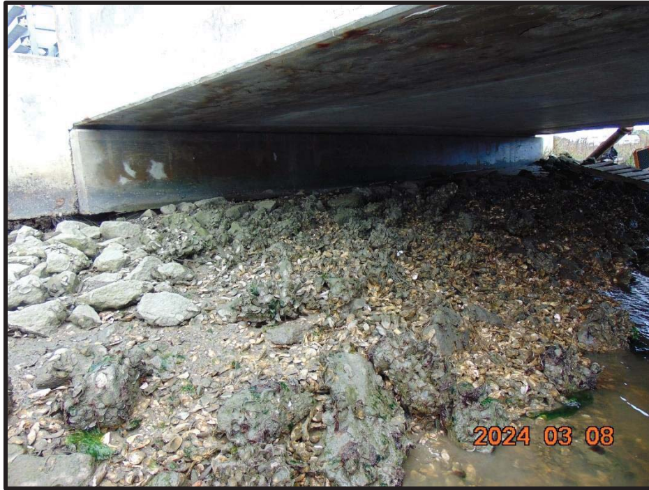
Photo 17: Bent 4 (Looking Upstream), Abutment 2
