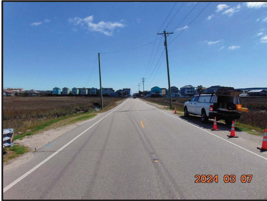
Photo 5: Roadway Approach from Bridge (Looking Southeast)
