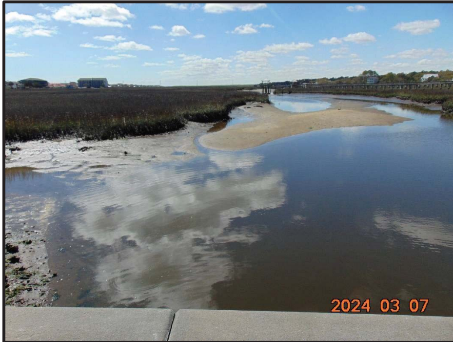
Photo 11: View From Bridge Deck (Looking Downstream)
