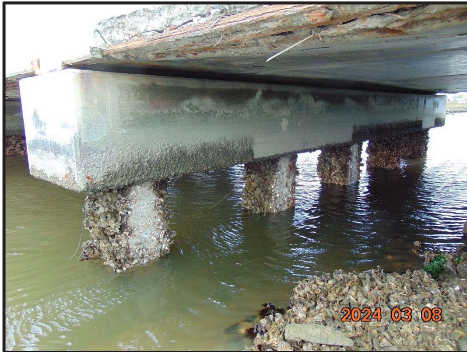
Photo 15: Bent 2 (Looking Upstream)
