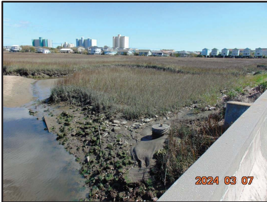
Photo 9: View From Bridge Deck (Looking Upstream)
