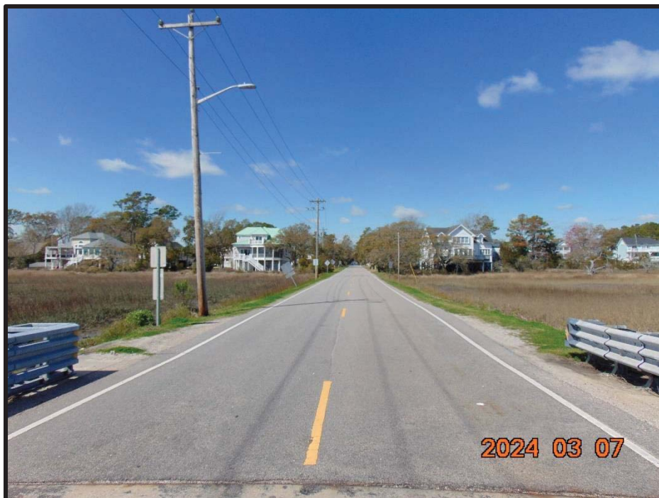
Photo 4: Roadway Approach from Bridge (Looking Northwest)
