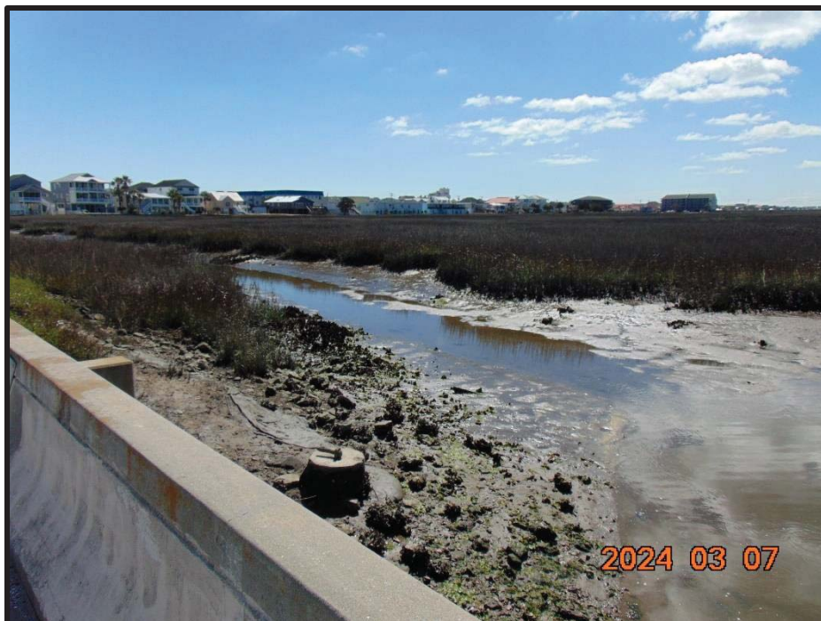
Photo 10: View From Bridge Deck (Looking Downstream)
