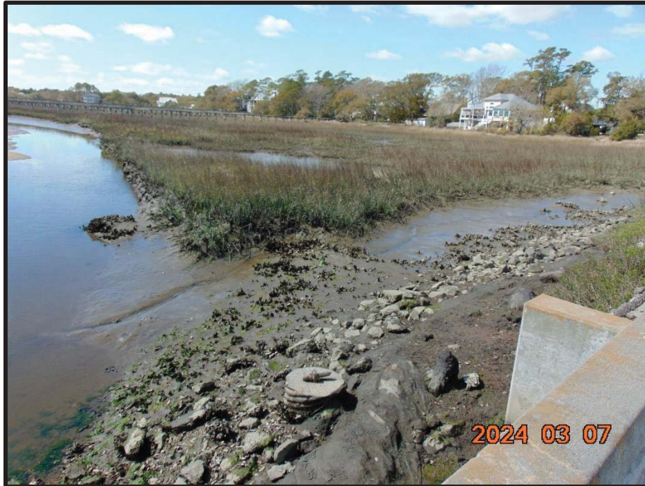
Photo 13: View From Bridge Deck (Looking Downstream)
