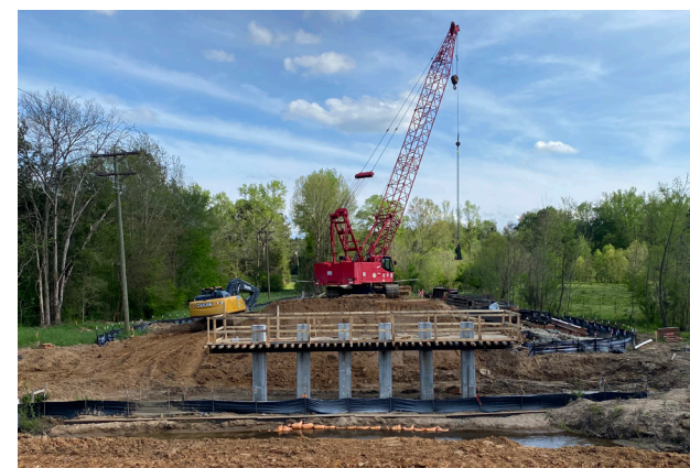
Cap and End Bent Construction - Graham Road
