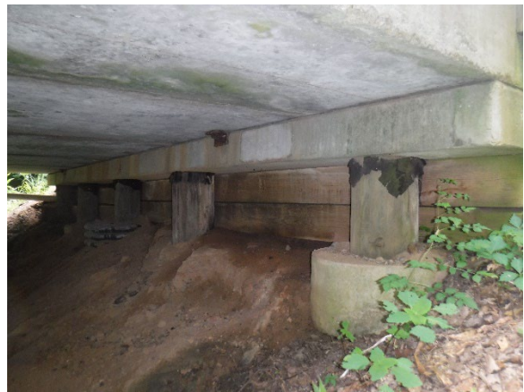
Photo 4. Timber Pile Cap Felt.
