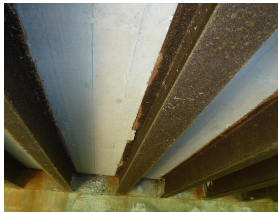
Photo 6 Underside View of Bridge Deck and Beams.
