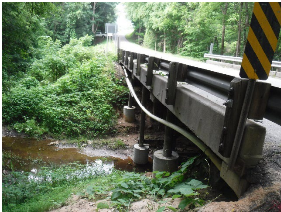
Photo 3. Southeast Side View of Bridge with attached Conduit.
