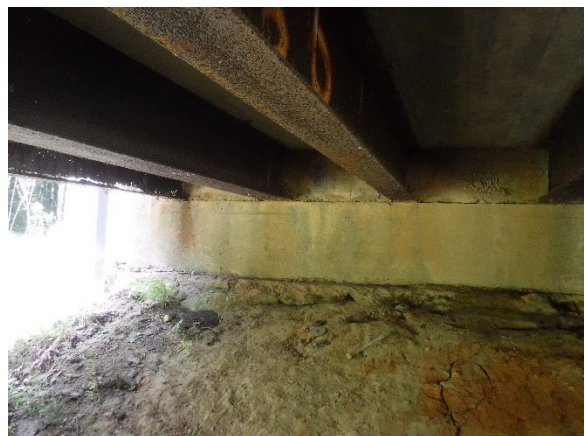
Photo 6. End Bent Associated with Bridge.
