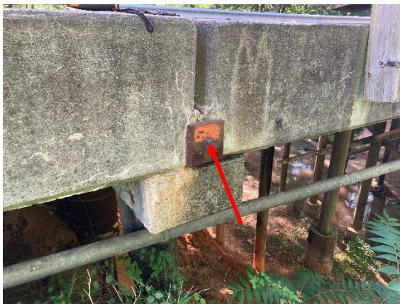
Photo 5. LBP on Orange Tie Rod Washers.
