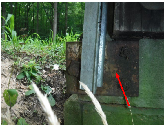
Photo 5. LBP on Orange Tie Rod Washers.
