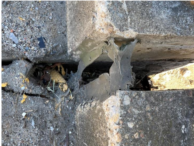
Photo 5: HA #2E and HA #2W Putty expansion joint (05779 + 05784)
