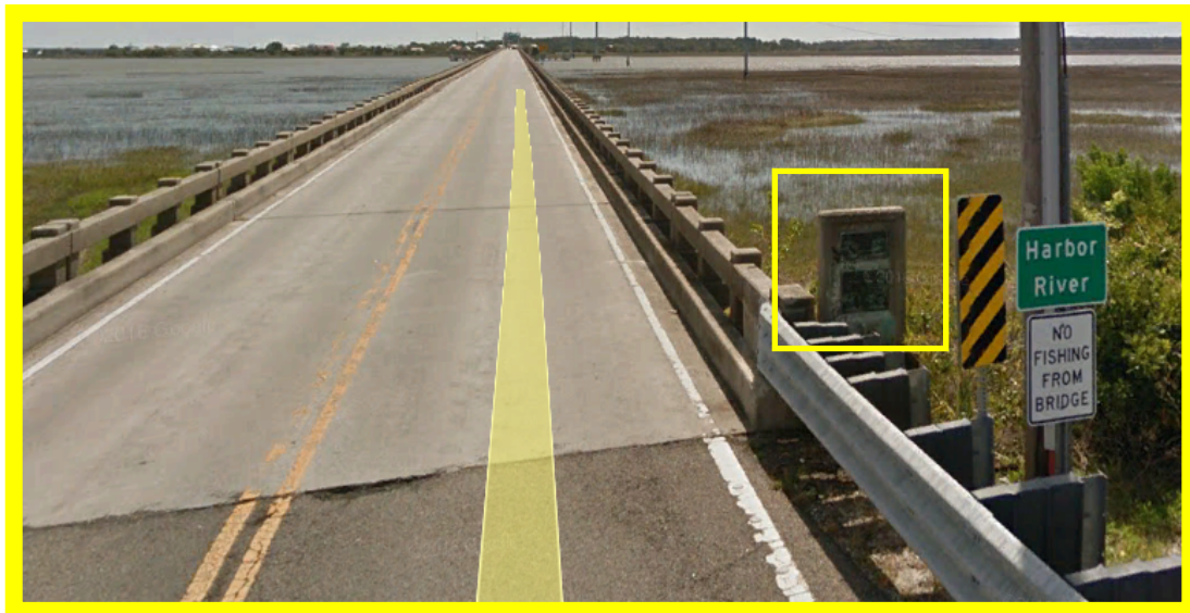
Bridge Placard Outlined in Yellow
