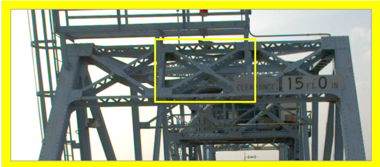
Section of Steel Cross Member Outlined in Yellow
