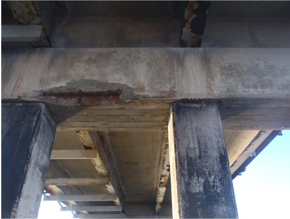
Photograph 11. Spall with 4 in. of penetration on the cap at Bent 56.
