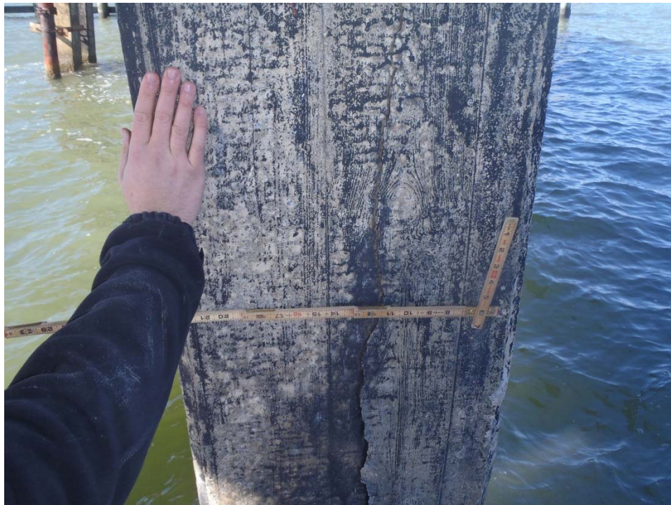
Photograph 10. 1/4-in. wide vertical crack in Pile 2 at Bent 45.
