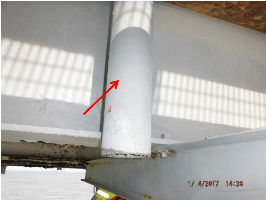
Bridge scupper pipes
