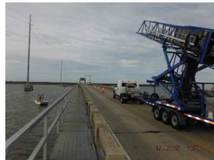
Photo 1 – Top view of SC-21 Bridge over Harbor River.
