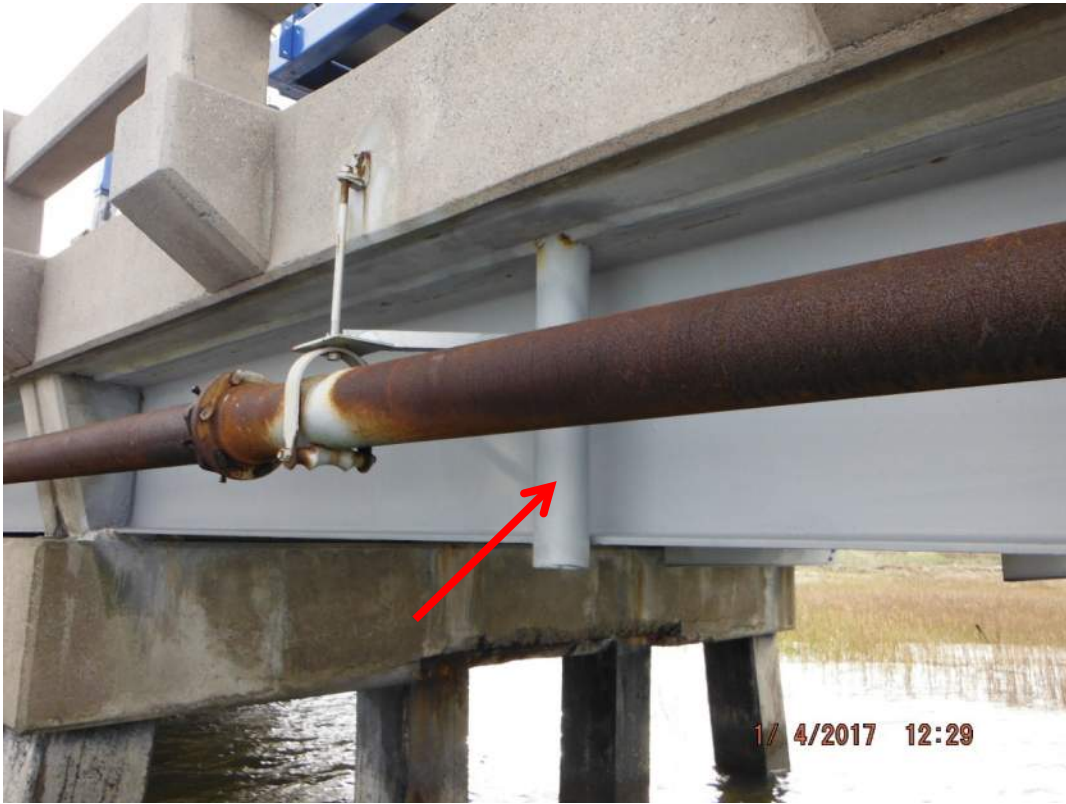
Bridge scupper pipes
