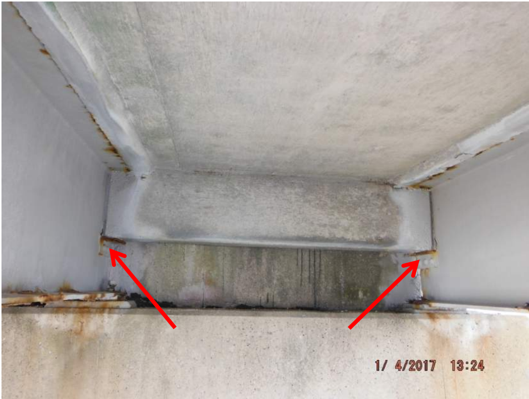
Bridge beam to diaphragm angle iron brackets
