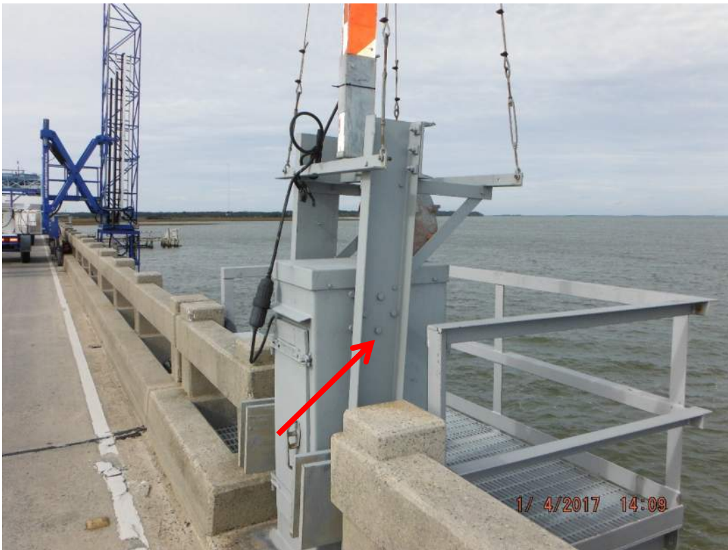
Bridge traffic control arm frame
