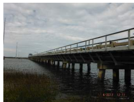
Photo 2 – Side view of SC-21 Bridge over Harbor River.
