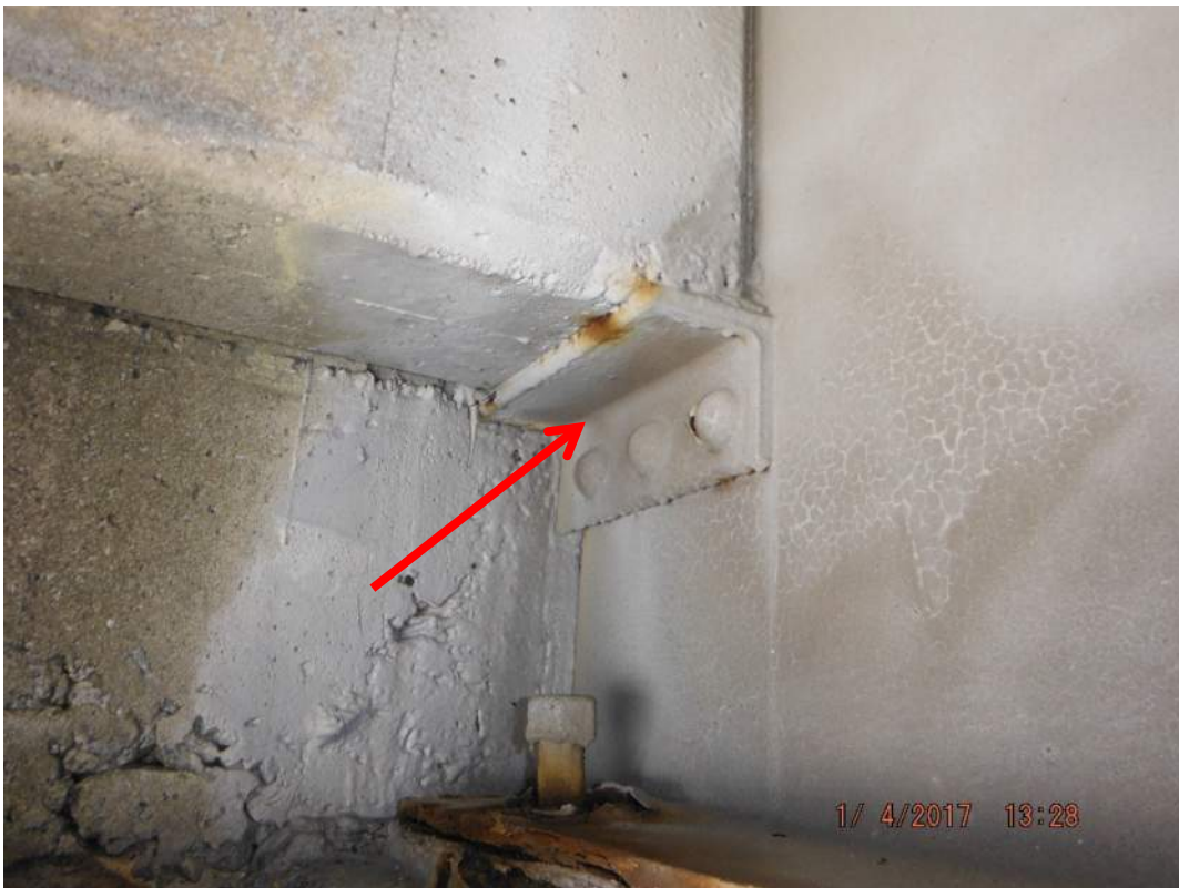
Bridge beam to diaphragm angle iron brackets
