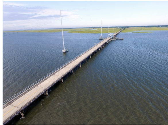
Photo 1 – US Highway 21 over the Harbor River.
