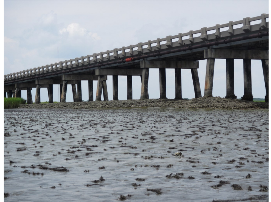
Photograph 12. Oyster beds formed around and between the existing piles for the US 21 Harbor River Bridge.
