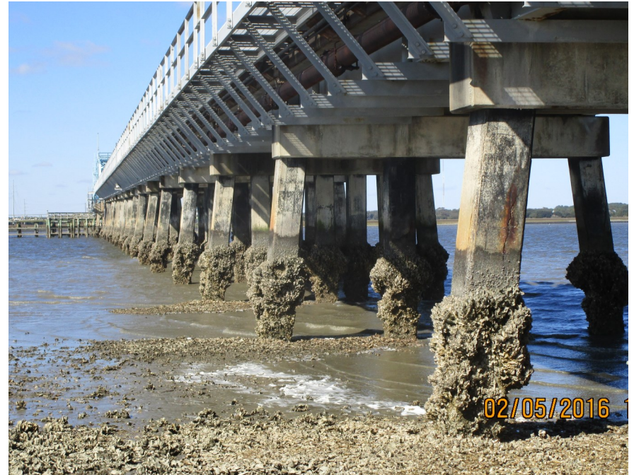
Photograph 18. Oyster shells encrusted on the existing US 21 Harbor River Bridge pilings on the eastern side of the bridge.
