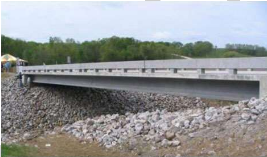
Figure 26: Single Span Bridge
