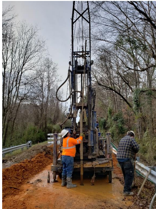
Drill rig on B-2
