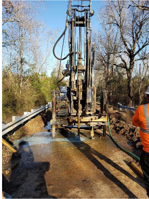
Drill rig on B-1
