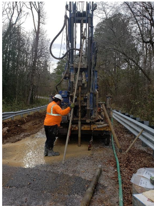
Drill rig on B-2
