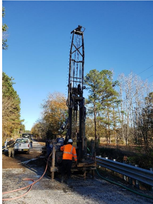
Drill rig on B-1
