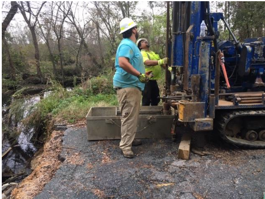
Drill rig on B-2
