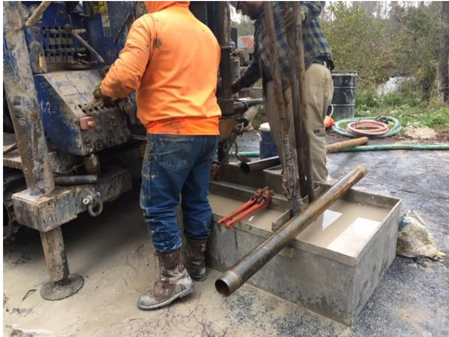
Drill rig on B-1
