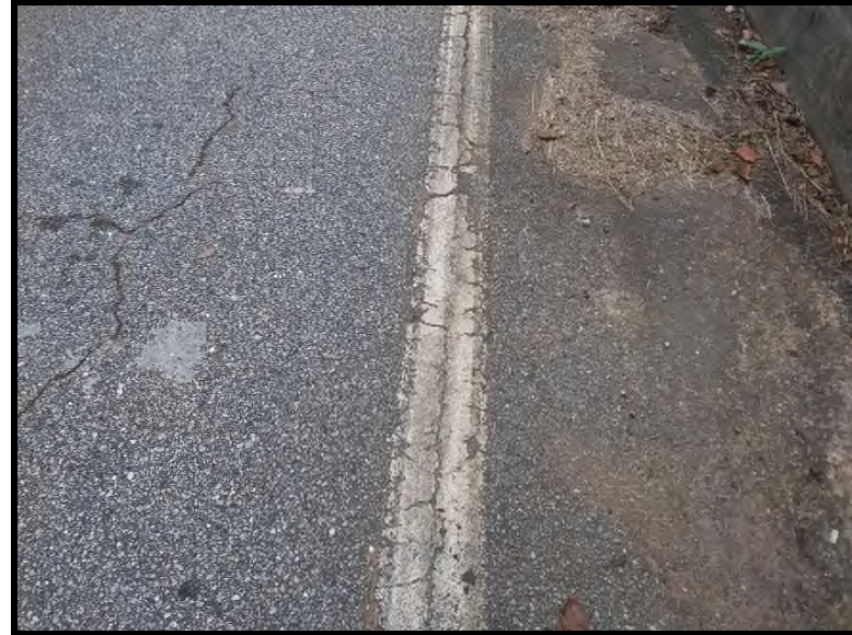
2 White stripes tested negative for lead-based paint.
