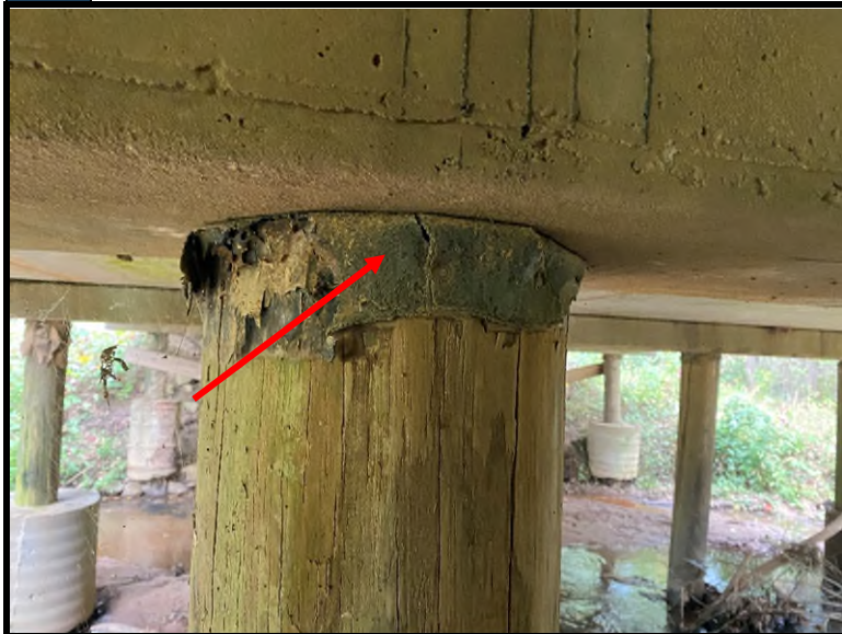
3 Felt paper tested negative for asbestos.
