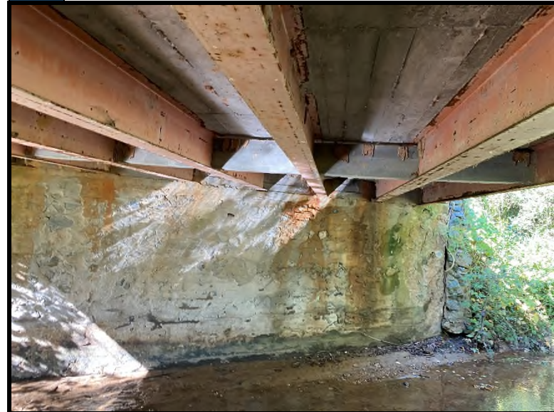
4 Orange I-beams tested positive for lead-based paint (7.30-10.1 mg/cm 2 ).
