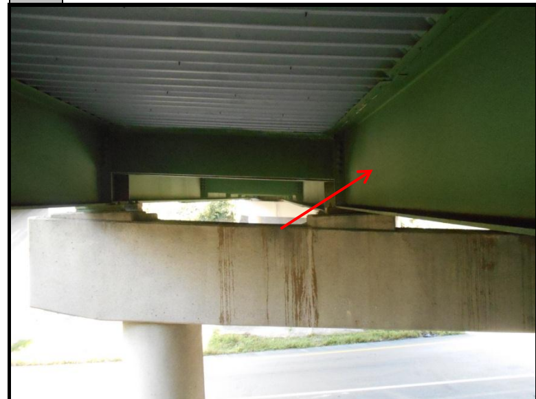
4 The green paint on I-beams tested positive for lead-based paint (0.8 mg/cm 2 ).
