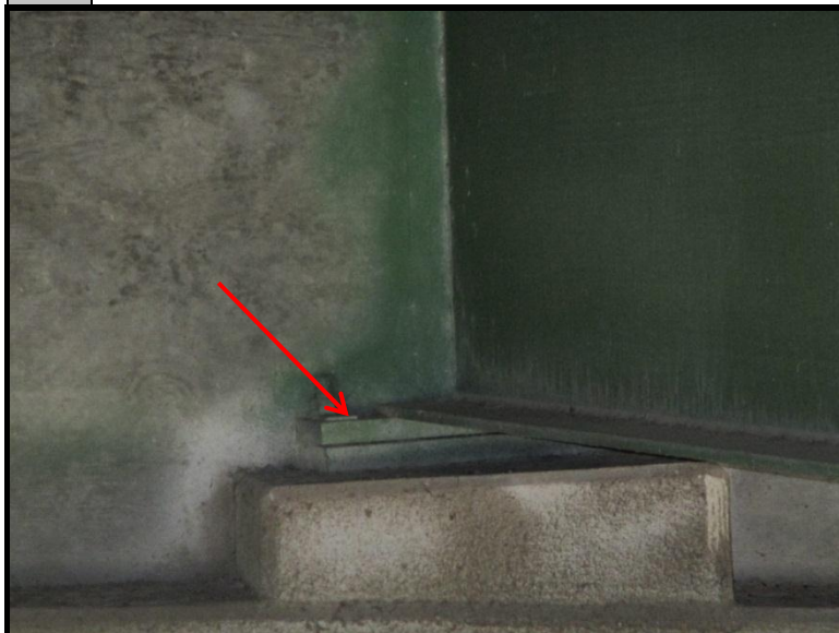
3 The green paint on the bolt plate tested positive for lead-based paint (0.8-2.0 mg/cm 2 ).
