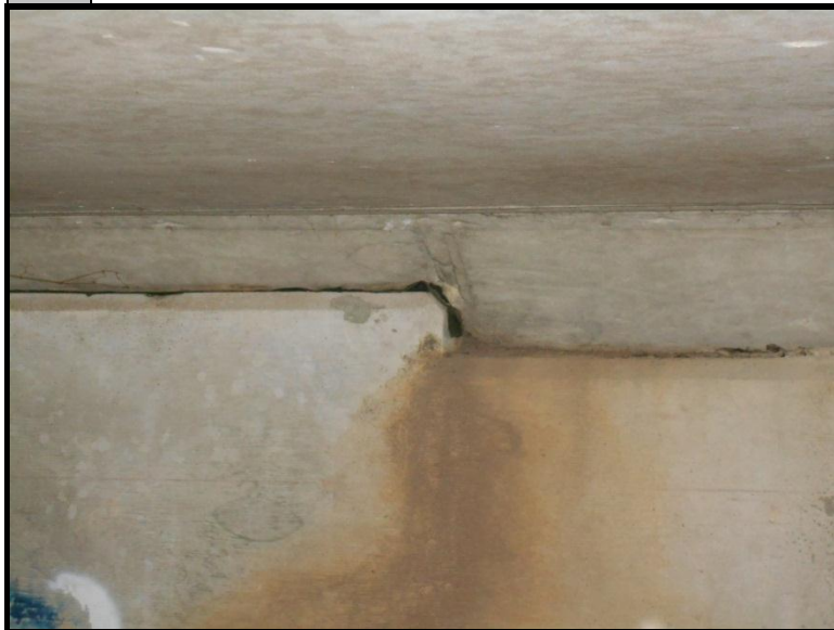
3 View of the tar paper associated with the I-77 bridges over Windsor Lake. The tar paper tested negative for asbestos.
