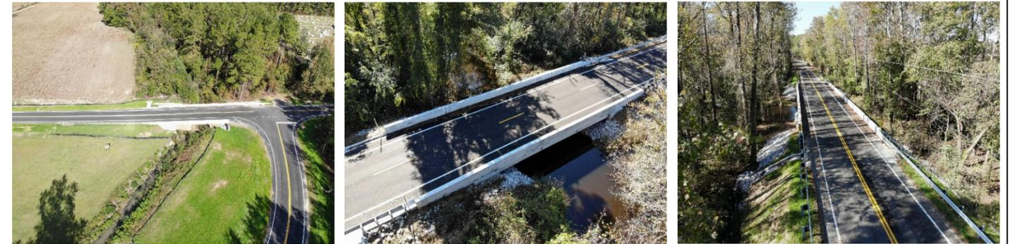
**S-51 over unnamed creek (left photo):** 70’ single span bridge on 15 degree skew. End bents utilized steel pile foundations, superstructure consisted of 24” cored slab units with AWS. Adjacent intersection was reconstructed as part of the project.
