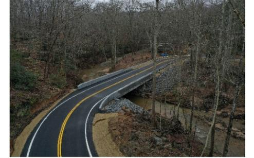
This includes recovering from a second flood, immediately post award, that changed the site and scope of work at S-174. The existing bridge completely collapsed during the second flood, and embankment material leading up to the bridge was washed away. The roadway embankment, and slope protection had to be recreated prior to completing the bridge replacement.
