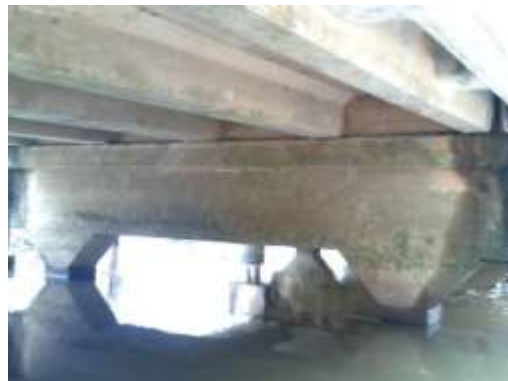
PHOTOGRAPH 06 UNDER BRIDGE VIEW
