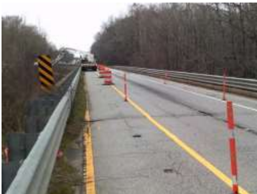
PHOTOGRAPH 05 BRIDGE TOP VIEW
