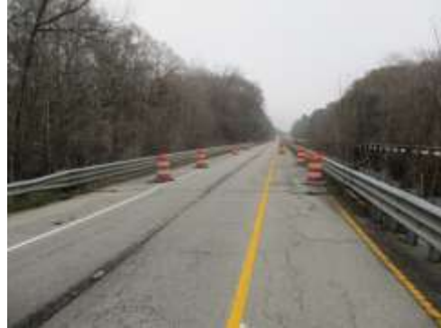
READING # 10, 11, 12 TYPICAL TRAFFIC PAINT/ GUARD RAILS (WEST BOUND LANES )
