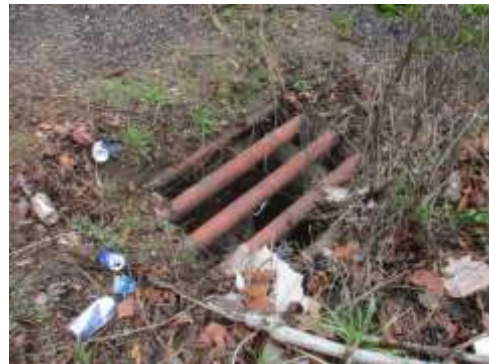
READING # 7, 14 TYPICAL METAL STORM DRAIN GRATE
