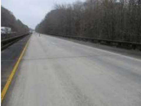
READING # 4, 5, 6, TYPICAL TRAFFIC PAINT/ GUARD RAILS (EAST BOUND LANES )
