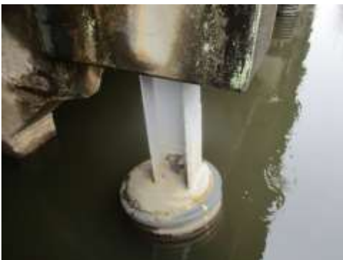
READING # 15 TYPICAL BRIDGE METAL SUPPORT COLUMN
