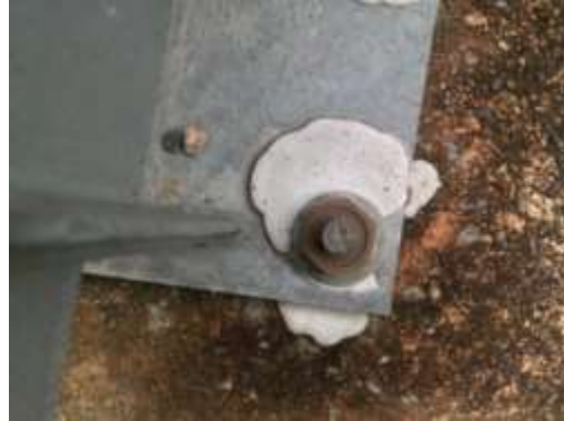
HOMOGENEOUS AREA 02 GUARD RAIL MASTIC (GRAY)
