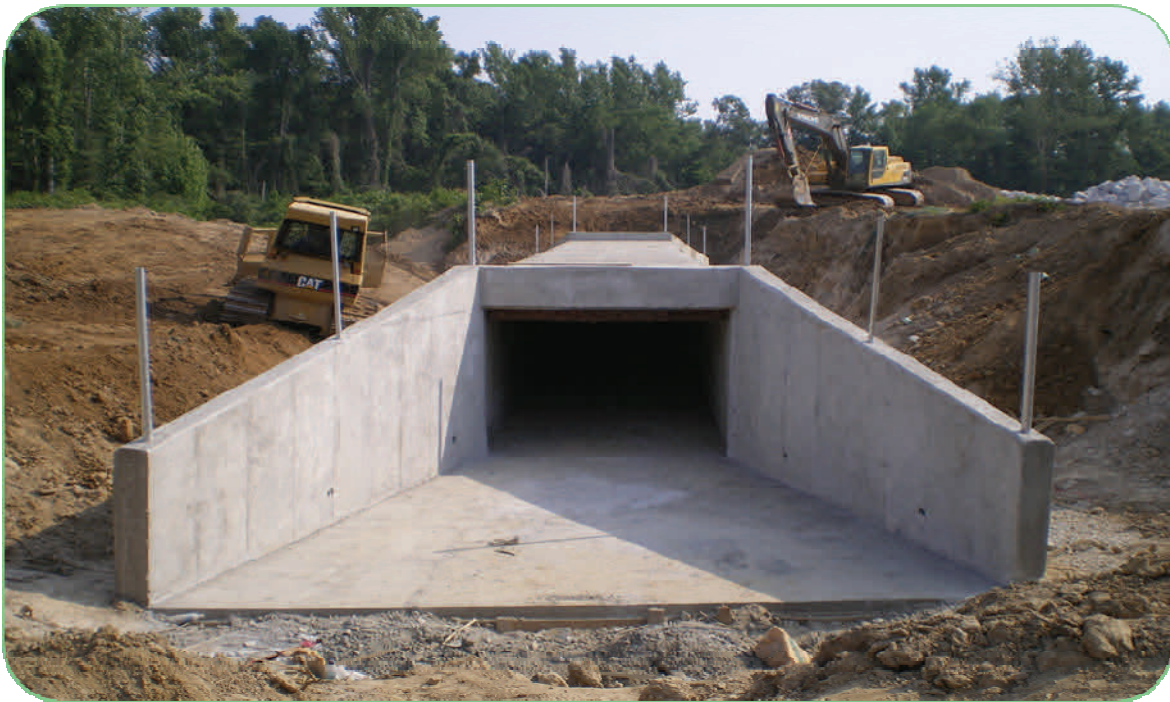
New Box Culvert with flared end and concrete apron
