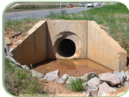
RCP with headwall and wingwalls
