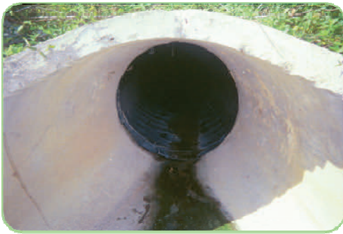
HDPE pipe with flared concrete end section
