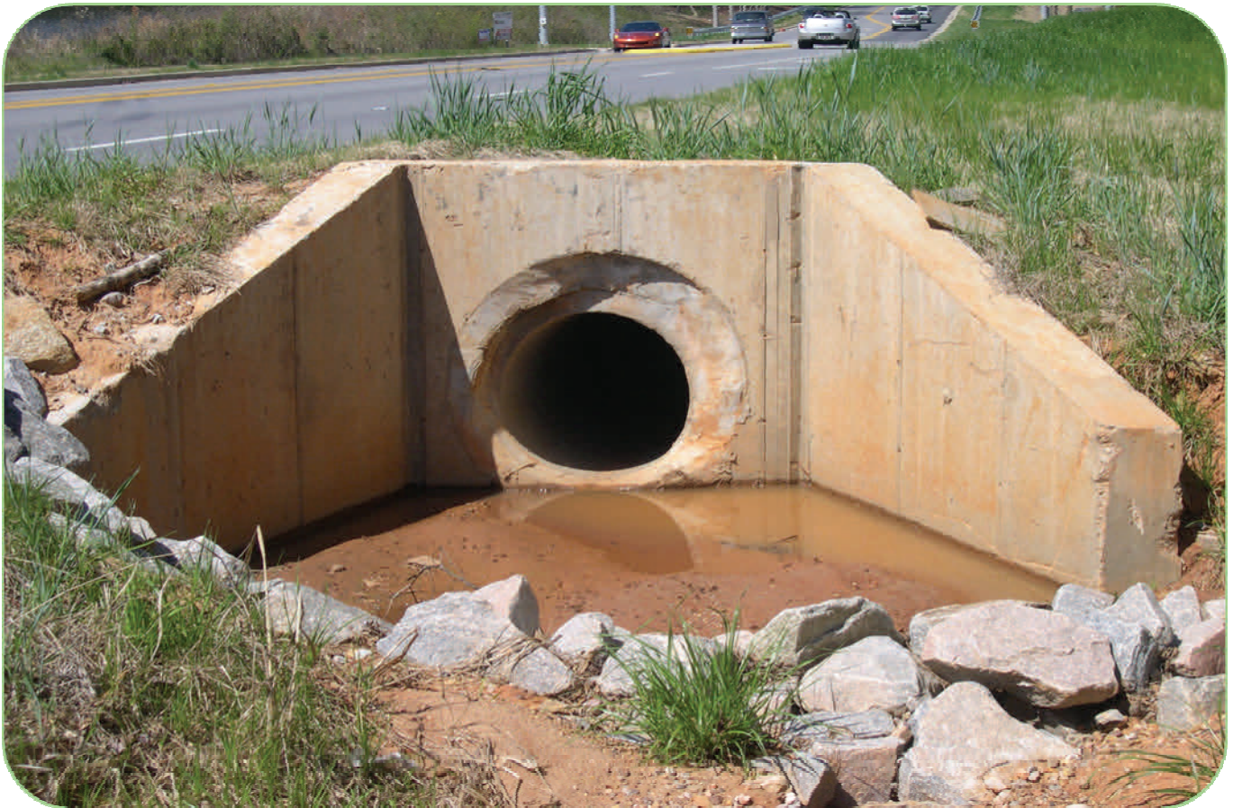
Headwall and Wingwalls with Rip Rap
