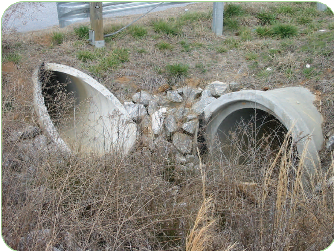
Beveled End on the left and Flat End on the right
