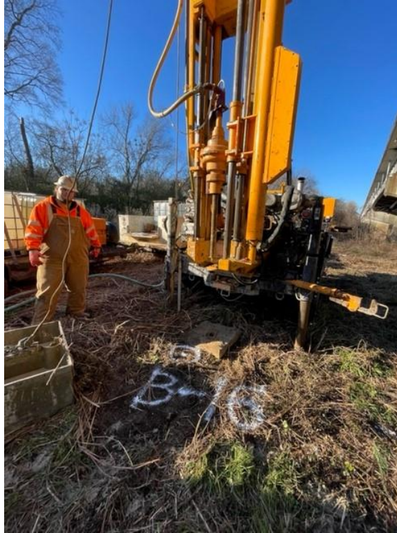
Drill rig on B-16
