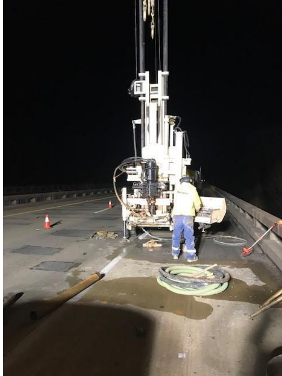
Drill rig on B-14
