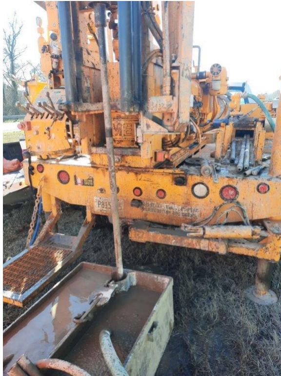
Drill rig on E-5
