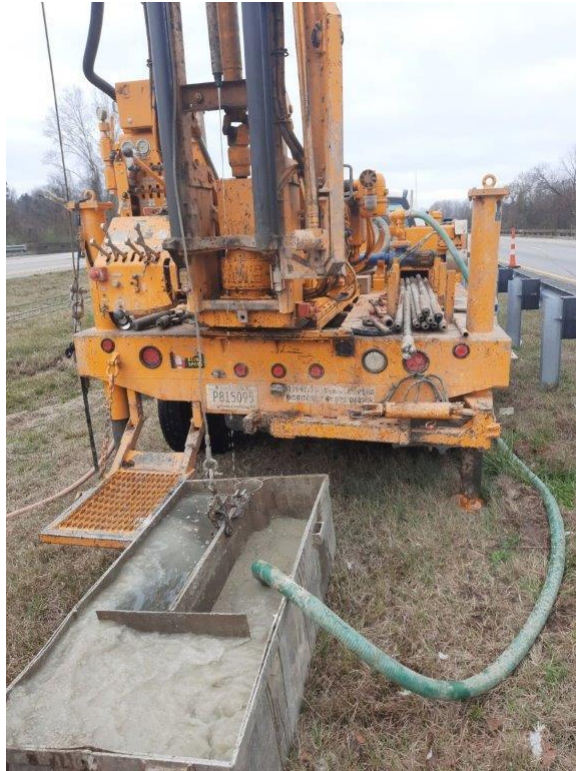
Drill rig on E-4
