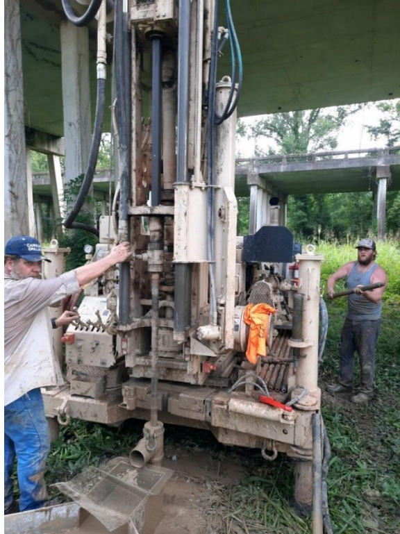
Drill rig on B-3
