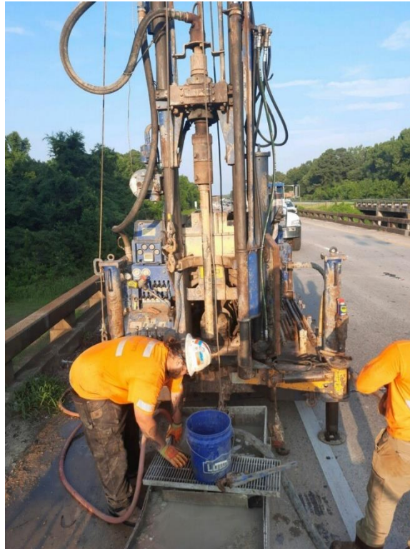
Drill rig on B-1
