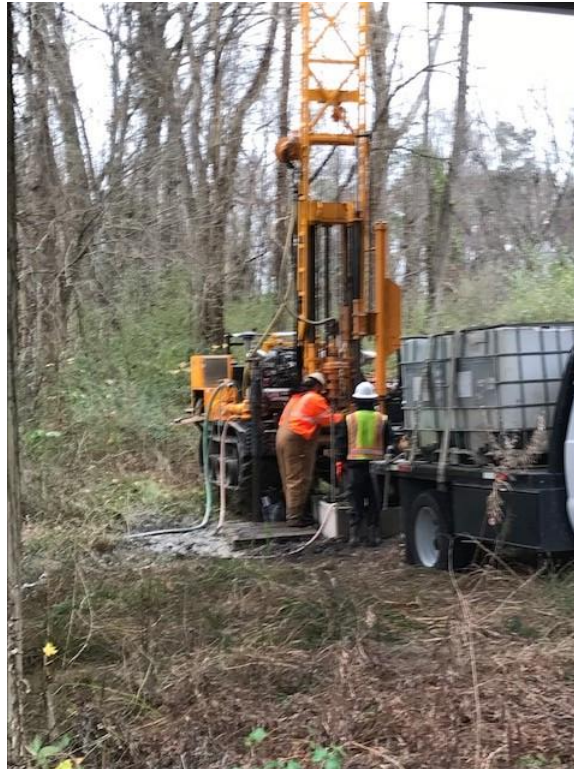
Drill rig on B-10
