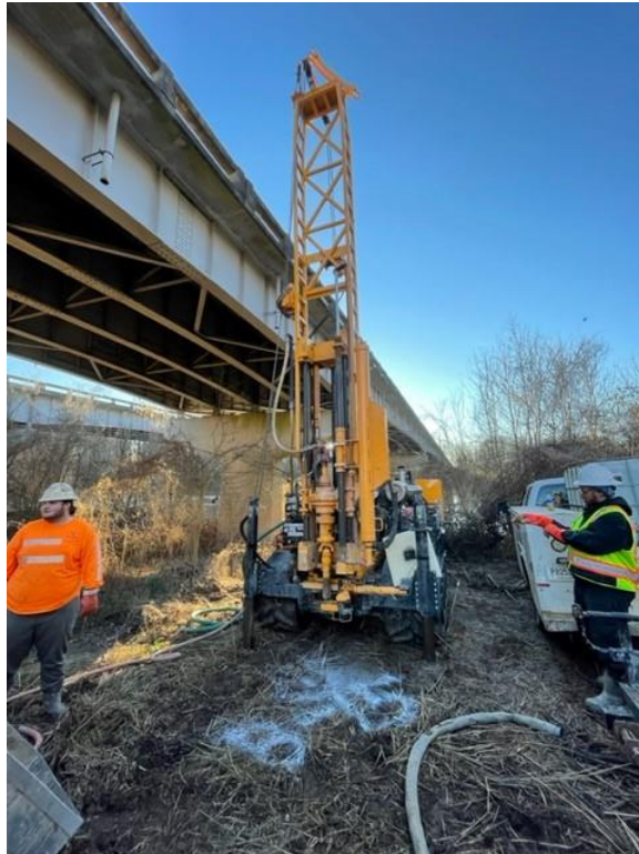
Drill rig on B-15
