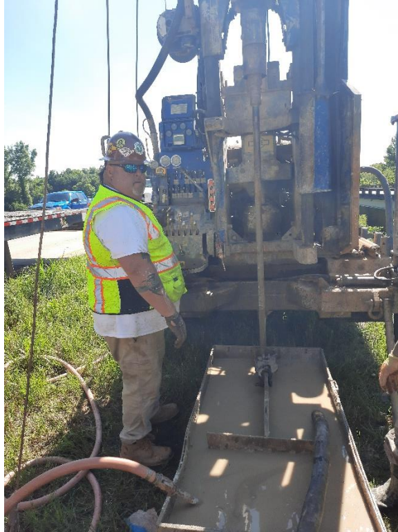
Drill rig on B-9
