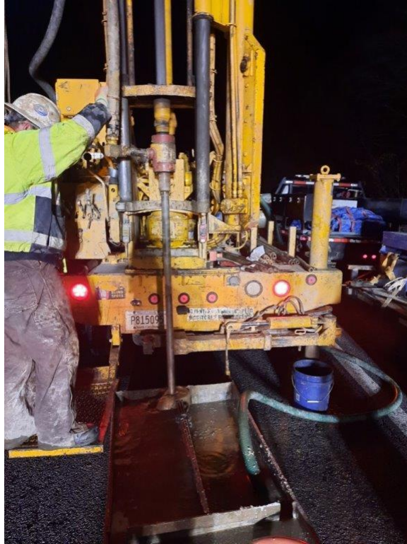
Drill rig on R-9
