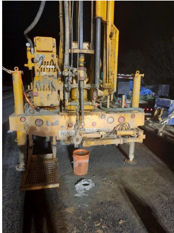
Drill rig on R-5
