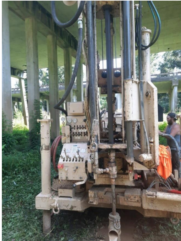
Drill rig on B-4
