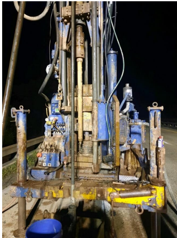
Drill rig on B-2
