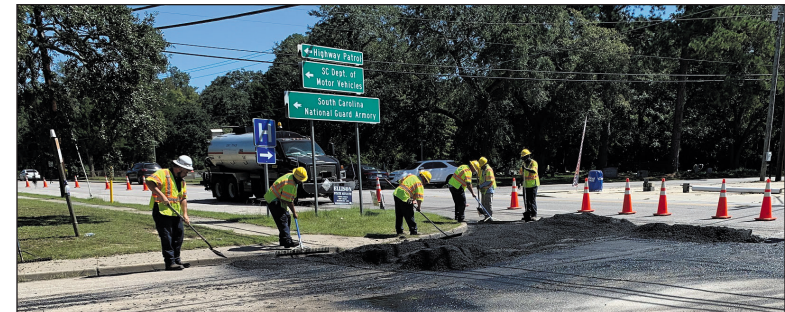
Crews level the asphalt at the intersection.
