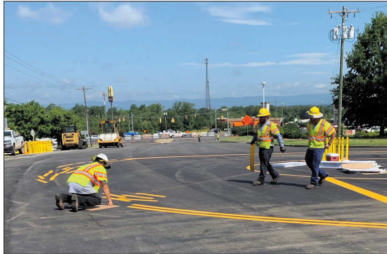
District 3 Maintenance workers, from left, Charlie Orsborne, Chris Wilson and Randy O'Connor lay out the traffic pattern for a new roundabout in Travelers Rest.
