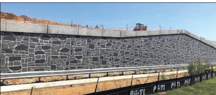
The project also included the replacement of two stone retaining walls.
