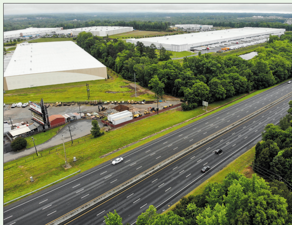
The new interchange will be Exit 81 in Rock Hill.
