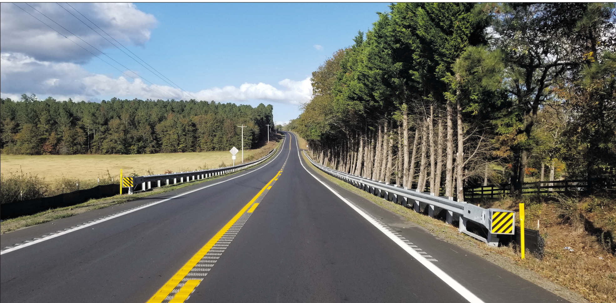
BOBBY USRY/AIKEN CONSTRUCTION
