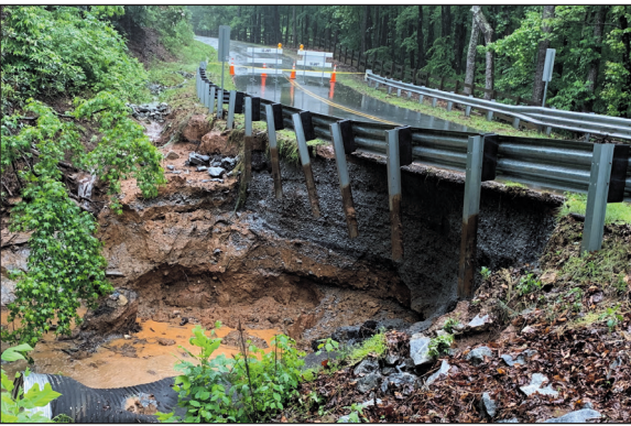
BEFORE: Dug Hill Road
