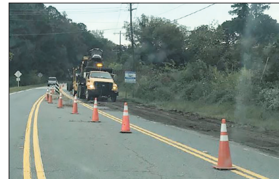
Crews do shoulder regrading in Chester County.
