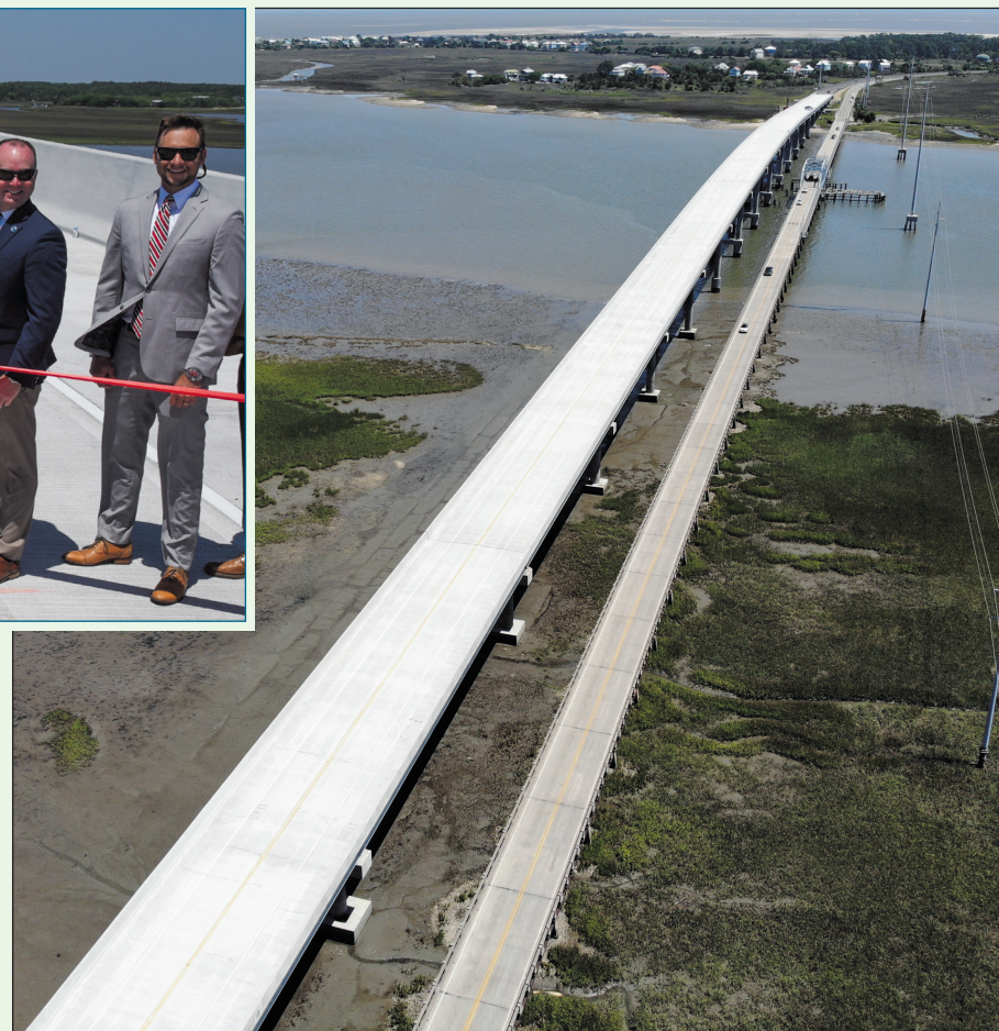
The new bridge is 3,350 feet long and rises 75 feet above the river. It will replace the old Sea Island Parkway swing span.
