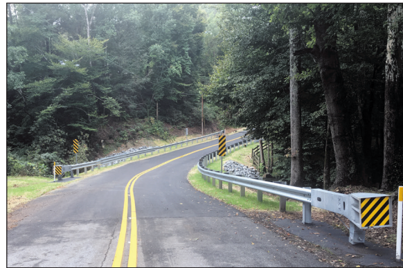
AFTER: Dug Hill Road
