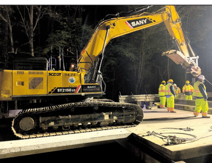
An excavator removes slabs from the interior spans.
