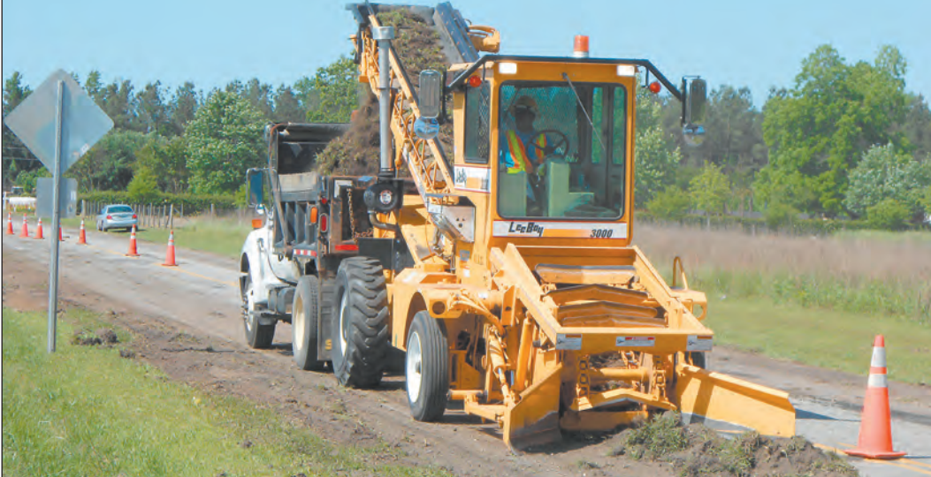
Kingstree Maintenance employee Jessie Mack operating the Lee Boy unit as Mosel Wilson follows along with the dump truck, as the crew takes advantage of the beautiful spring weather to clean shoulders in the county.
