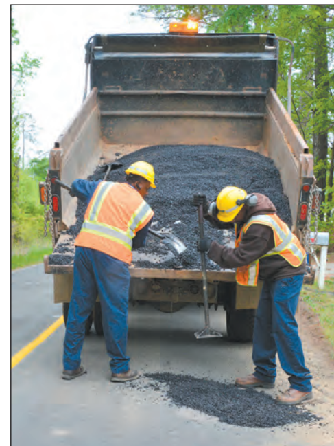
ABOVE and RIGHT: Richland Maintenance crews sweep and make patching repairs along Old Bluff Road, the detour route for Bluff Road in Richland County.
