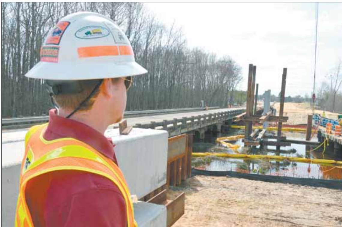
Robert Griffin of Florence Bridge Construction supervises the drilling of bridge pilings over Lake Swamp as part of the widening project of U.S. 76 near Timmonsville. The project widens 3.75 miles of U.S. 76 and associated side roads to accommodate the new alignment.
