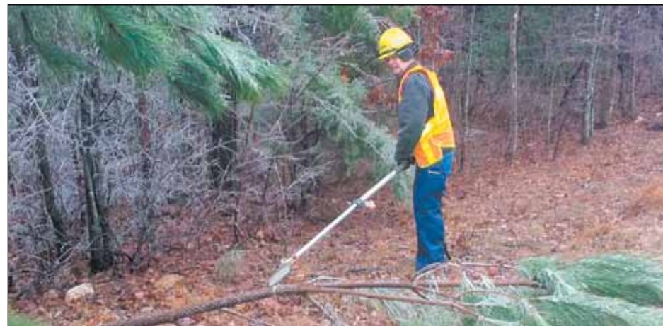
PHOTO BY JAMES CATOE/KERSHAW MAINTENANCE
