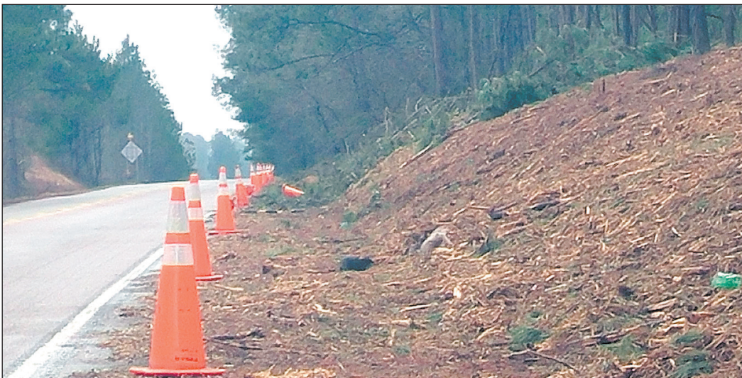
The District's vegetation clearing improves motorists views down the highway and also gives a cleaner shoulder should vehicles leave the road.
