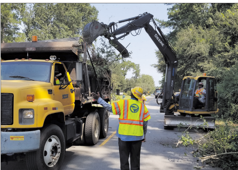
Crews remove debris along S.C. 61 after the storm.
