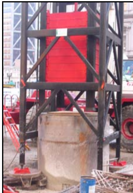
Figure 24-5, High-Strain Load Testing Apparatus (GRL Engineers, Inc.)
