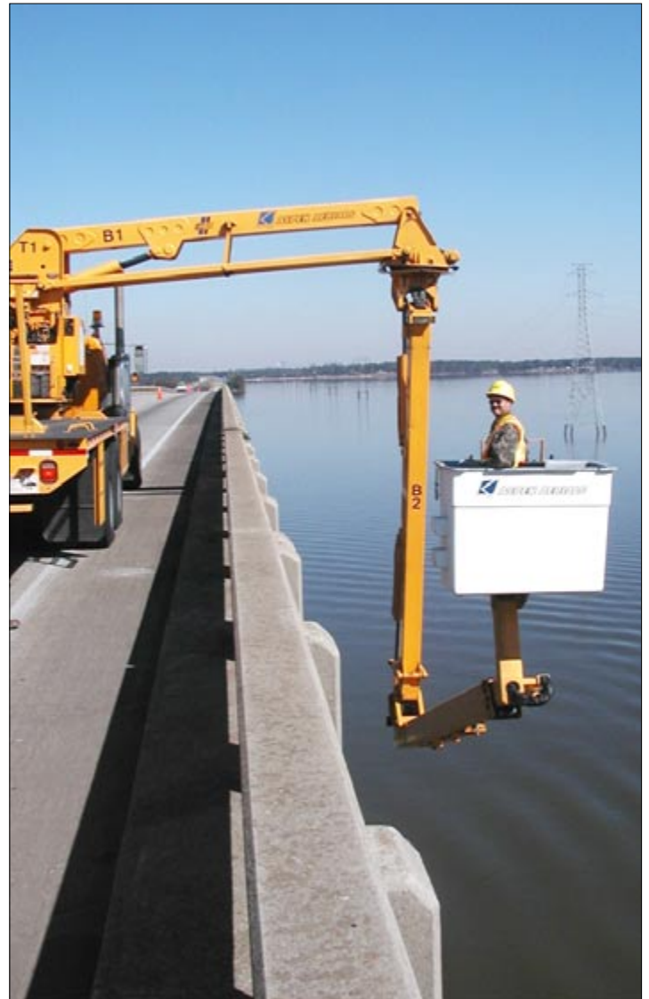
VAN D. WALTERS/DISTRICT 7 BRIDGE INSPECTION
