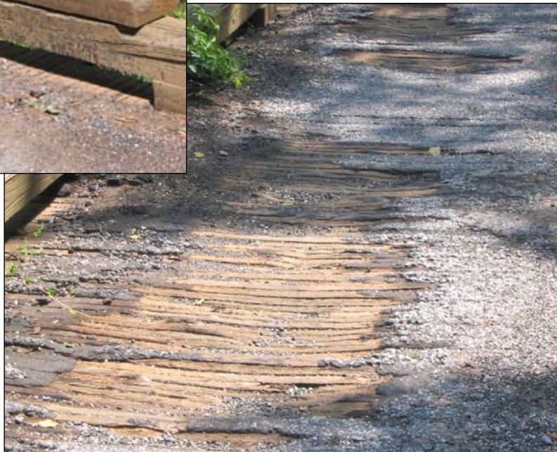
Here, wood can be seen under the thin layer of asphalt on the old roadway.
