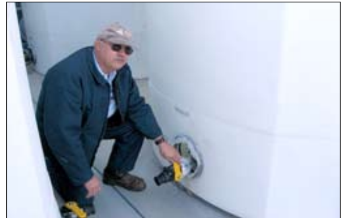
PHOTOGRAPHS BY EDWARD MOORE/DISTRICT 4 Mac Mobley checks on snow plow equipment and the salt brine tanks at Rock Hill Maintenance.
