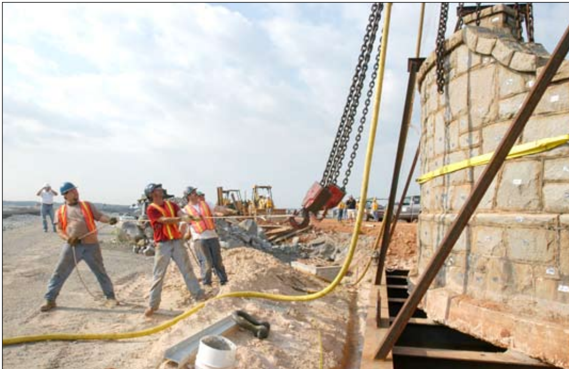
Workers unhook and remove heavy chains and hooks after one of the stone gates was moved.
