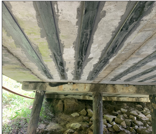
Carbon fiber strips applied underneath certain bridges can fix weight load restrictions.
