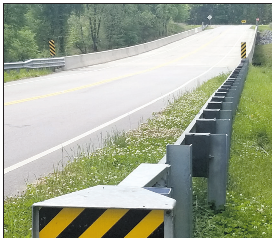
York County Bridge on Auten Road
