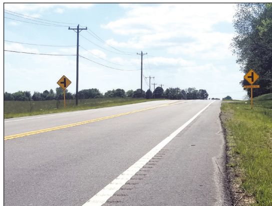
Highway 72 near Chester after repaving and safety improvements
