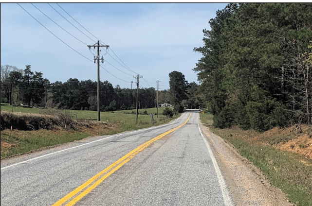
This image shows a cement reclaimed base with chip seal membrane.
