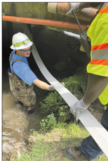
Carbon fiber strips applied underneath certain bridges can fix weight load restrictions.
