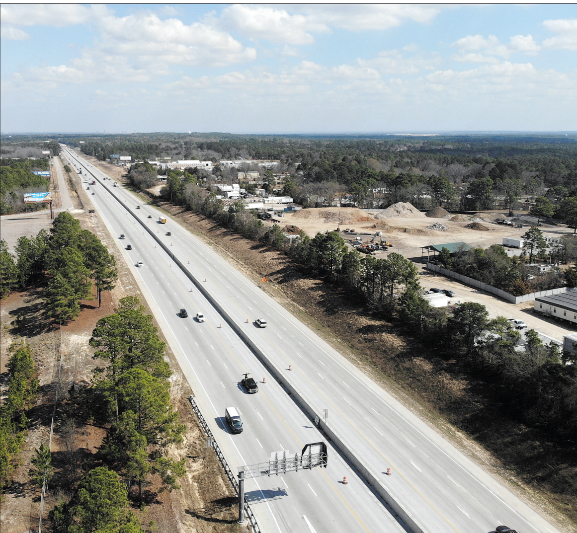
A newly widened section of I-20 is seen here with six travel lanes (up from four) on Feb. 24, 2022. The I-20 widening project is anticipated to be complete in June 2022. Photograph taken near the S.C. 6 / I-20 interchange in Lexington County.
