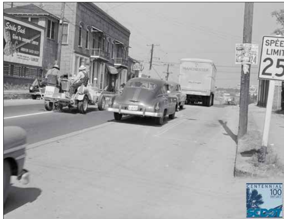
Highway Department maintenance forces mark the center line on U.S. 1 in West Columbia (going toward the Gervais Street Bridge) in April 1951.
