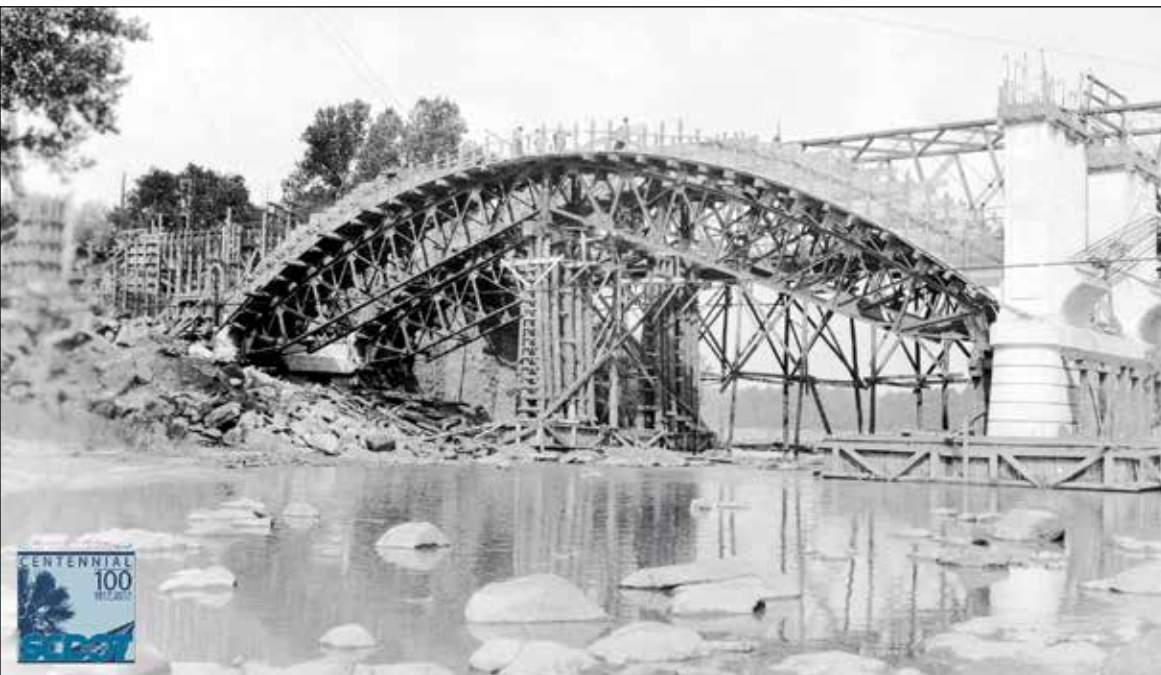
The Gervais Street Bridge under construction in Columbia in 1927
