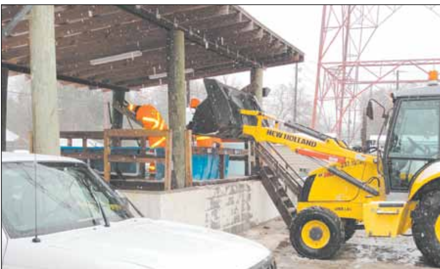
Darlington Maintenance prepares salt brine for spraying.
