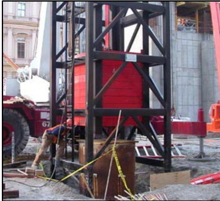
Figure 24-5, High-Strain Load Testing Apparatus (GRL Engineers, Inc. (2015))
