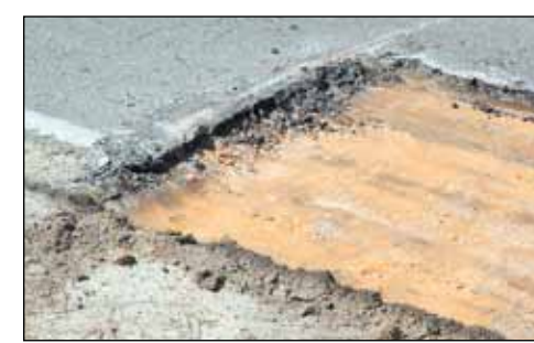
Due to the freezing, thawing and refreezing during the recent winter storms, sections of pavement were cracked and damaged. The affected highways are patched using full-depth patching where pavement is removed to the base before being repaved with asphalt.
