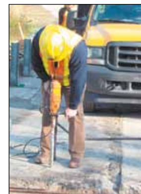
Chris Team uses a core drill on the bridge deck. The drill cuts through concrete and rebar.
