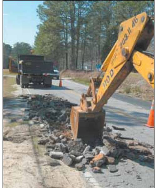
Due to the freezing, thawing and refreezing during the recent winter storms, sections of pavement were cracked and damaged. The affected highways are patched using full-depth patching where pavement is removed to the base before being repaved with asphalt.
