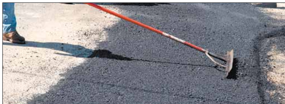
Due to the freezing, thawing and refreezing during the recent winter storms, sections of pavement were cracked and damaged. The affected highways are patched using full-depth patching where pavement is removed to the base before being repaved with asphalt.
