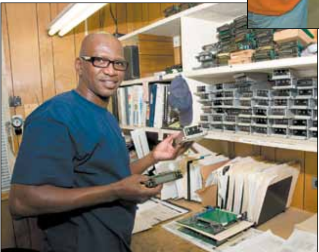
District 1 Traffic Engineering Technician Joe Butler checks loops detectors and load switches that go inside the signal control boxes.
