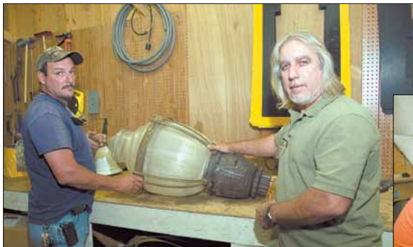
Mitchell Smith, left, and Ray Rast from District 1 work on a spare light head for the Blossom Street bridge. The lamp is a 250-watt high pressure sodium light that makes it glow yellow.
