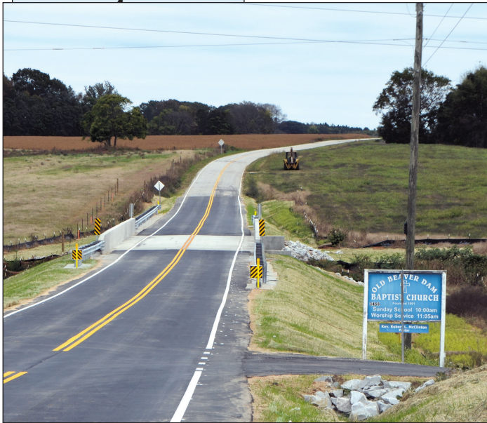
District 2 recently completed a bridge over Beaver Dam Creek on Beaver Dam Creek Road as part of SCDOT's 10-Year Strategic Plan.
