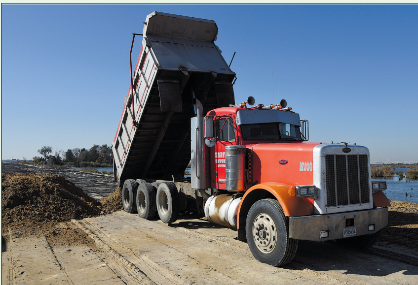
Borrow material is unloaded and soon to be spread at the U.S. 17 widening project in Jasper County on Dec. 2, 2021. This material is the first of a few different layers of material placed underneath the future riding surface.
