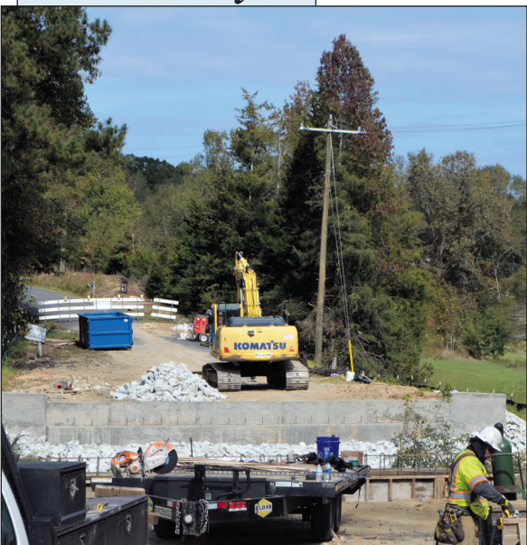
District 2 is replacing the bridge on Ridge Road over Camp Creek.
