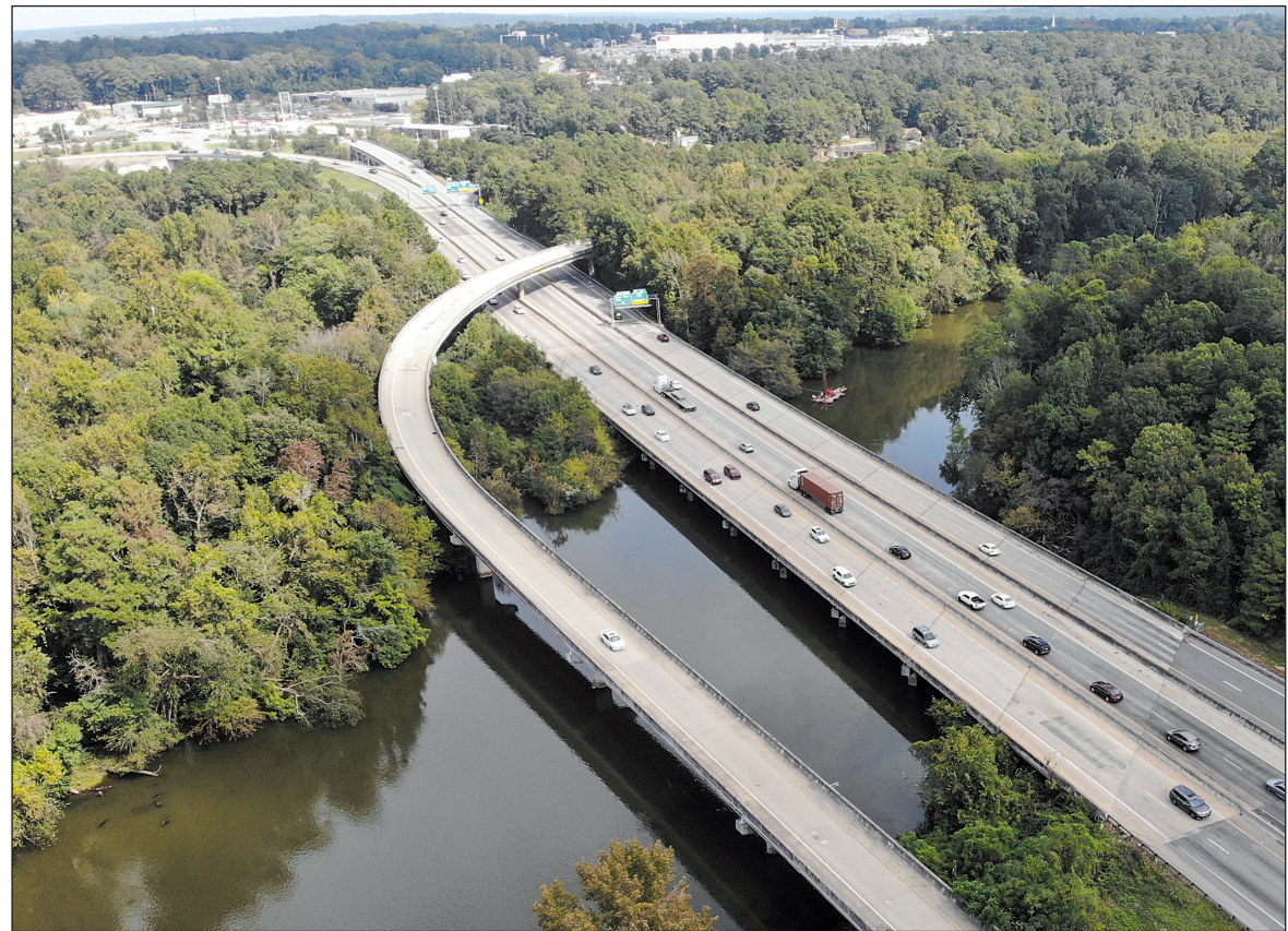
Phase 1 of the Carolina Crossroads project includes reconfiguring the Colonial Life Boulevard interchange as well as making improvements along I-126 and I-26. Here, the I-26 bridges and the I-126 flyover exit ramp toward Charleston are seen spanning the Saluda River on Oct. 14, 2021.
