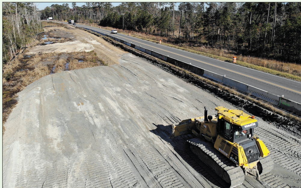
The borrow material is being spread by a bulldozer. As this road widening is built close to marshland, this material is one of many layers that are gradually built up to in order to properly drain water and support the future riding surface.
