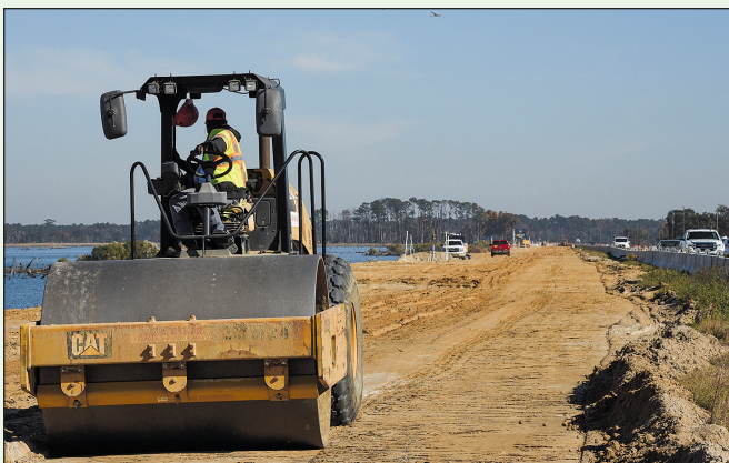
Borrow material is unloaded and soon to be spread at the U.S. 17 widening project in Jasper County on Dec. 2, 2021. This material is the first of a few different layers of material placed underneath the future riding surface.
