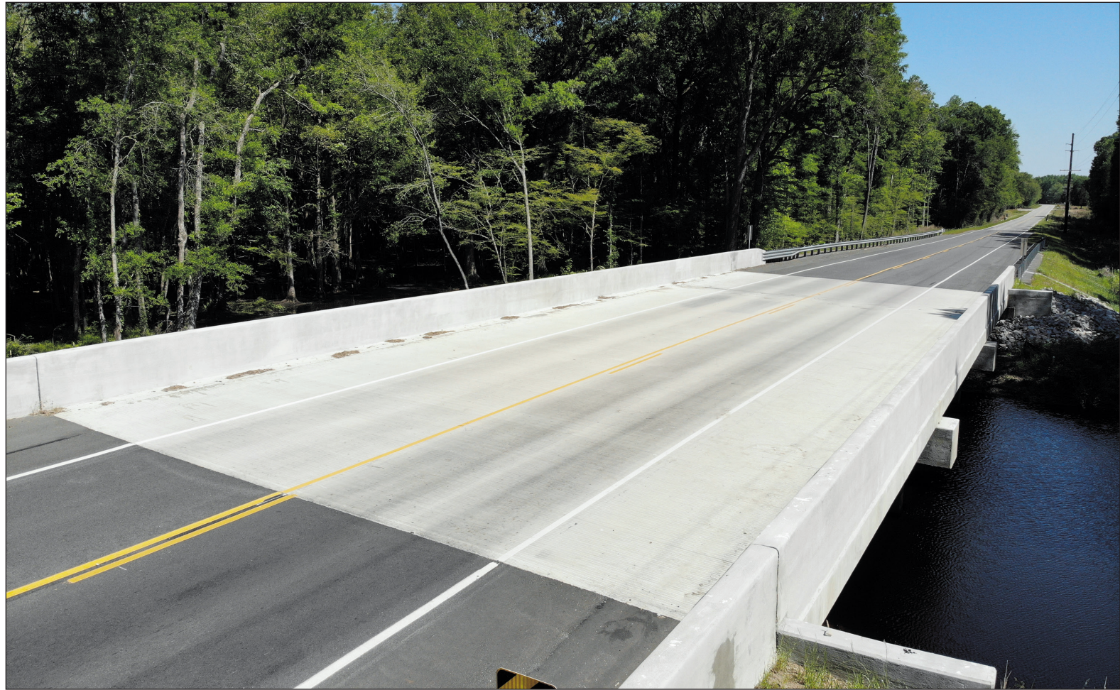
AFTER: The new bridge was constructed ahead of schedule in 111 days. A detour was in place for only 58 days. The new bridge is longer and wider than the bridge it replaced. This design-build project was recognized nationally for exemplifying the principles of design-build done right.
