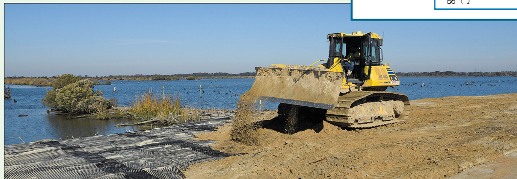
The borrow material is being spread by a bulldozer. As this road widening is built close to marshland, this material is one of many layers that are gradually built up to in order to properly drain water and support the future riding surface.
