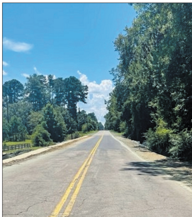
Aug. 12, 2021 - U.S. 17A - Repairs completed
