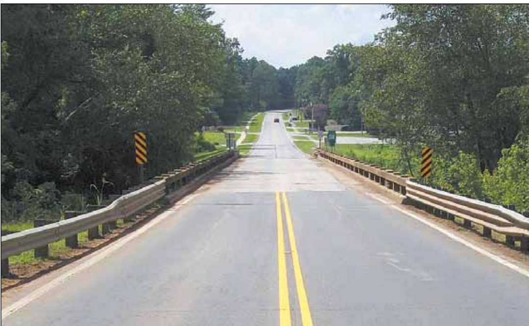
PHOTO BY FRITZ WEWERS/ANDERSON MAINTENANCE
