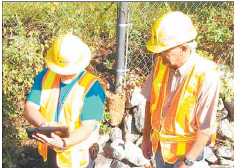
Tim Lisenby and Charles Stubbs use the iPad for culvert inspections using a server-based app.
