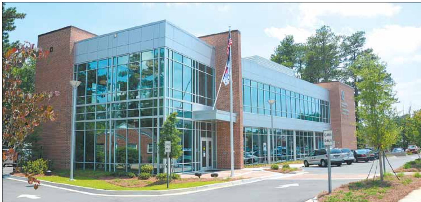
The new two-story, 9,150 square foot multi-modal transit facility and parking lot is the hub for the Cross County Connection public transit system in Orangeburg and Calhoun counties. The facility includes ticket sales, office space, conference rooms, passenger wait areas, drivers lounge, retail space and storage. The center is equipped with Internet, Wi-Fi and television for passengers.
