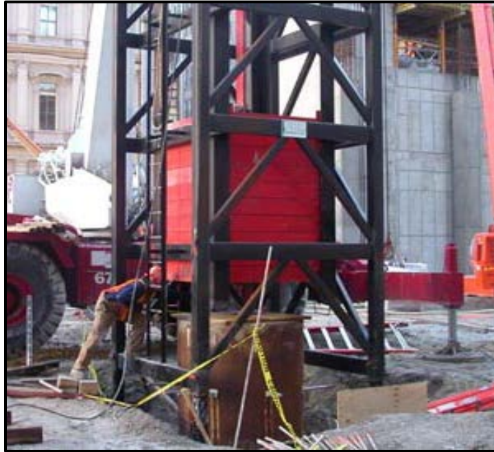
Figure 24-5, High-Strain Load Testing Apparatus (GRL Engineers, Inc. (2015))
